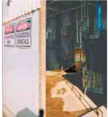
Chemical storage shed
