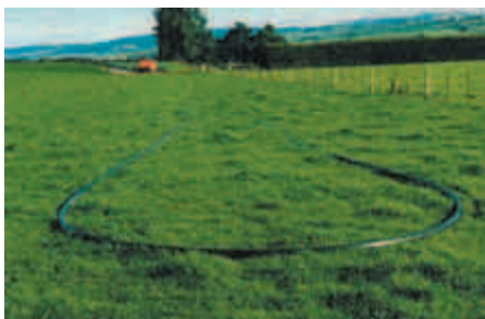
Pipe layout behind irrigator.
