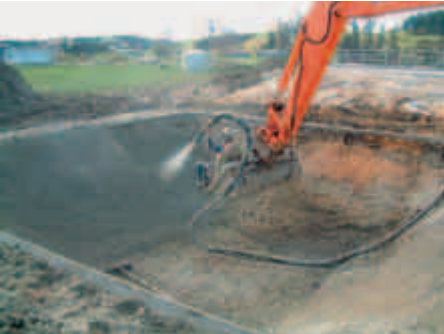
Concrete lining of a storage pond.
