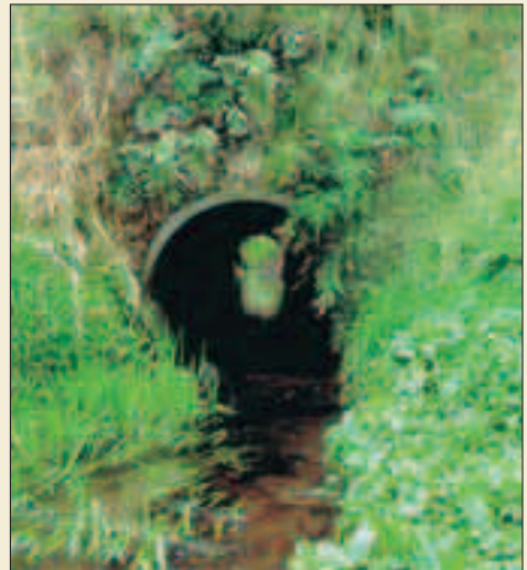
Well-designed culvert (level with bed, good fish access)
