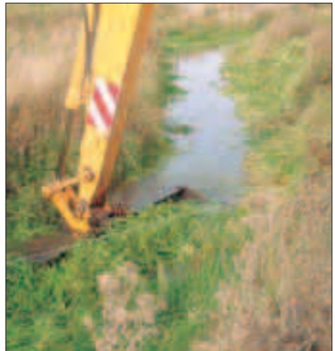
Keep drain banks less than 1:2 to maintain a fast flow in the channel
