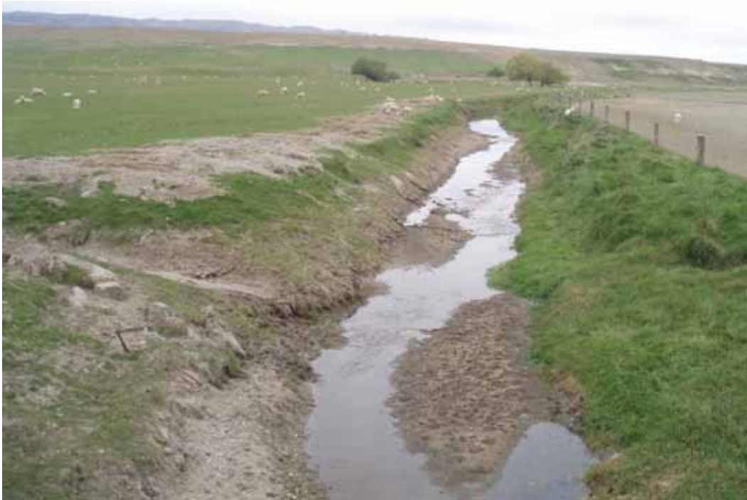
Figure 23. Pool Burn upper looking up from the Auripo Road bridge
