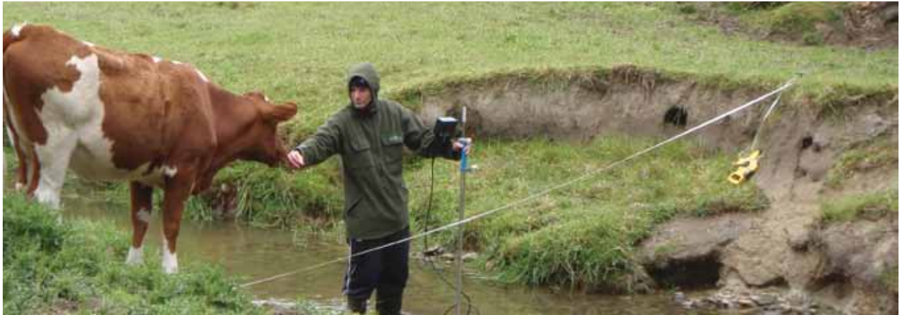
Figure 6 Possible source of sediment: bank collapse
