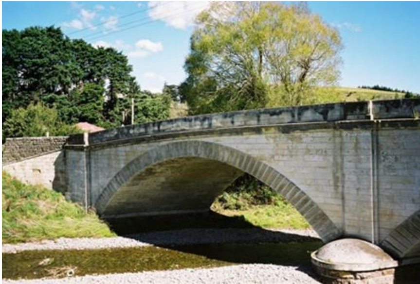
Figure 15. The historic Waianakarua Bridge, built over the North Branch of the Waianakarua River in 1874 (Image courtesy of Nicola Jackson, Heritage New Zealand Pouhere Taonga).
