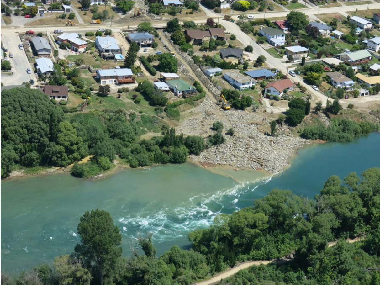
Figure 3.11 The Reservoir Creek debris fan the day after the debris flow event. There are two excavators in the photo, one at the SH8 bridge over Reservoir Creek and one on the lower fan clearing the concrete channel (Photo: Ben Mackey, ORC; 27/11/2017).
