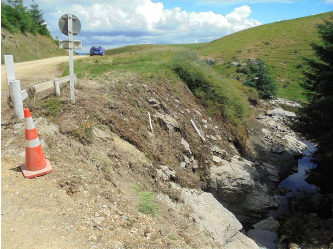
Figure 3.19 The small bridge over Tima Burn showing evidence for a large volume of water passing over the bridge, destroying posts and railings and stripping soil and pasture off the banks of the stream, exposing bare rock, rather than alluvium (Photo: S.Dellow 13/12/2017).
