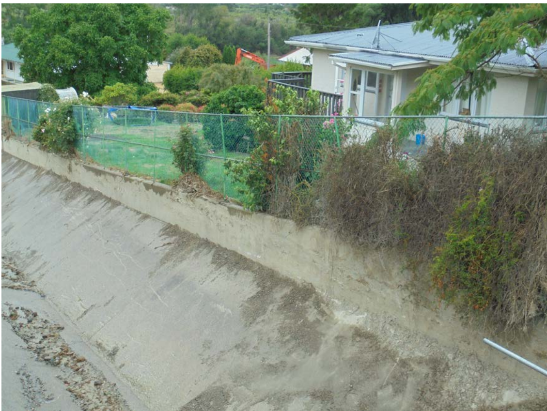
Figure 4.1 Undamaged fence on top of the concrete channel on the Reservoir Creek fan (Photo: S.Dellow 13/12/2017).
