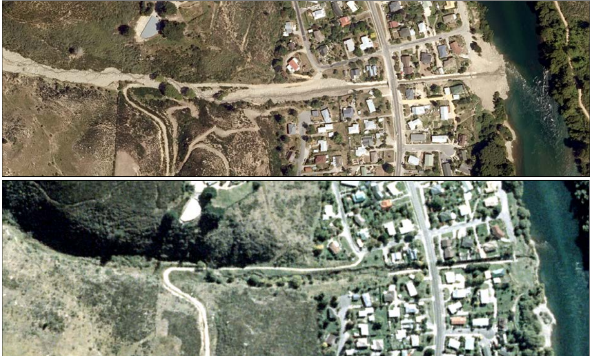
Figure 3.12 Before (bottom; 30 th March 2006) and after (top; 28 th December 2017) photos of the Reservoir Creek debris flows of 26 th November 2017. The debris is largely confined to the stream channel which stands in contrast to the 2005 Matata debris flows shown in Figure 2.1.
