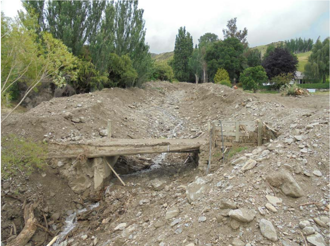
Figure 3.14 Pump Station Creek debris flow deposit at the farm bridge on the upper part of the debris flow fan (Photo: S.Dellow 13/12/2017).
