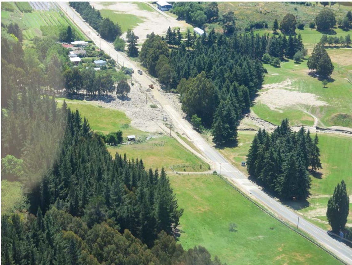
Figure 4.4 Debris blocking SH8 at Golf Course Creek has been cleared sufficiently to allow single lane traffic flow the day after the debris flows (Photo: Ben Mackey, ORC; 27/11/2017).
