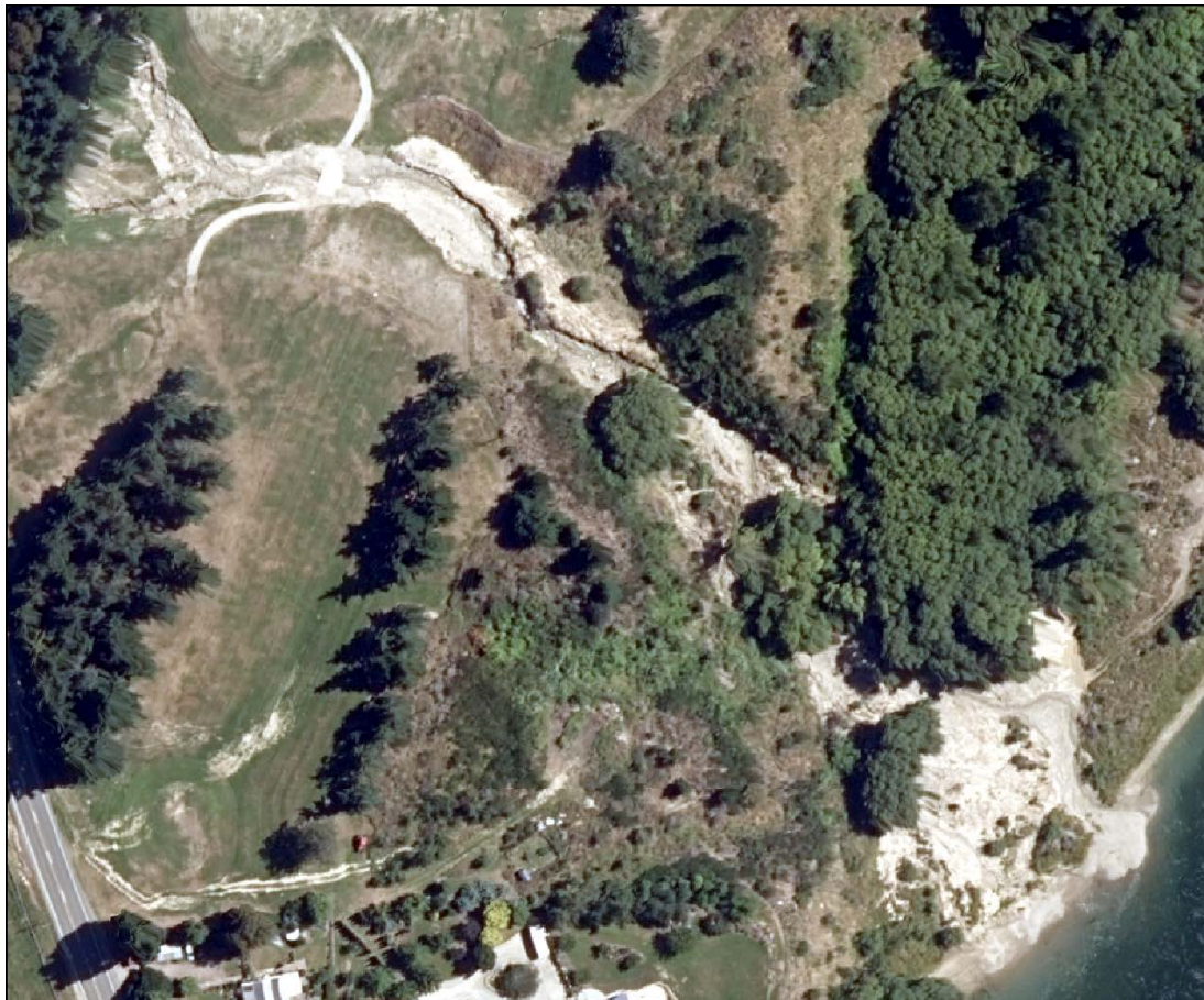
Figure 3.9 The creek bed between SH8 (left of the picture) and the Clutha River showing the results of scour and deposition on the Golf Course Creek fan (Photo: Aerial Surveys, 28 th December 2017).
