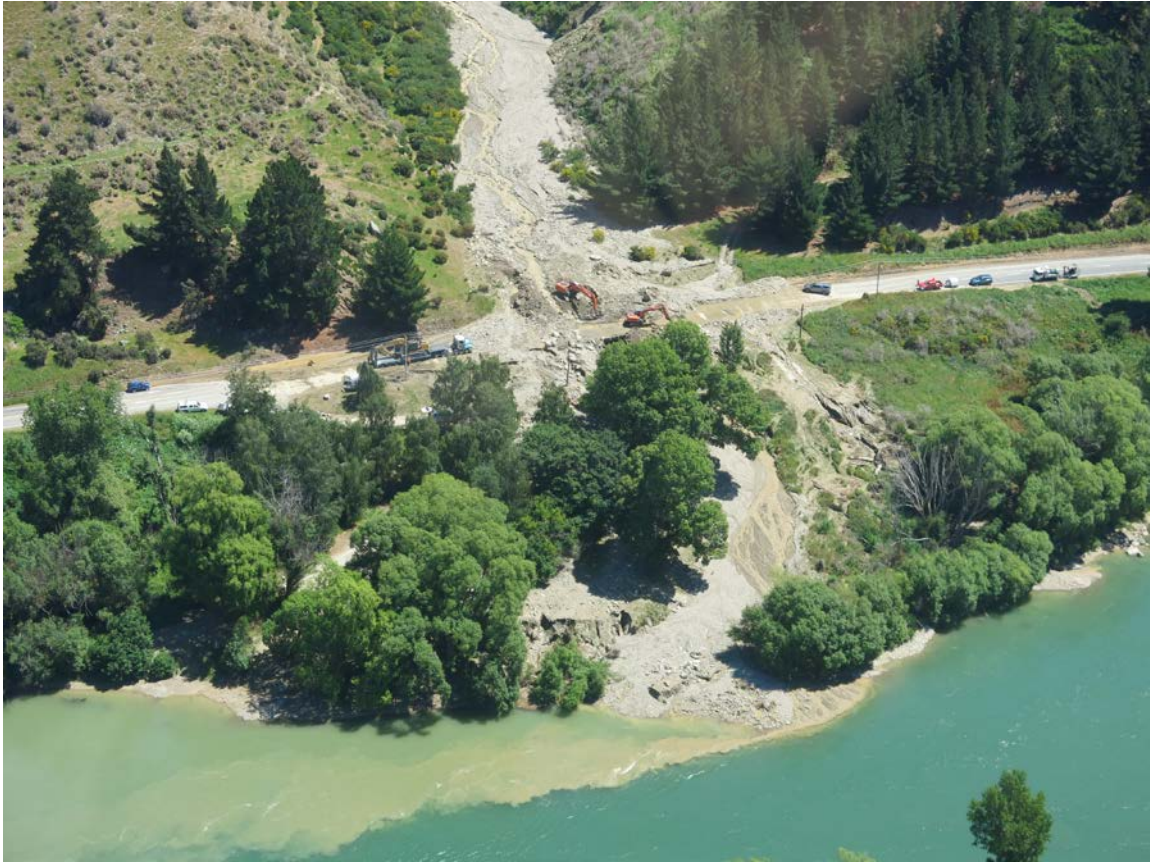
Figure 4.3 Debris blocking SH8 at Black Jacks Creek (Photo: Ben Mackey, ORC; 27/11/2017).
