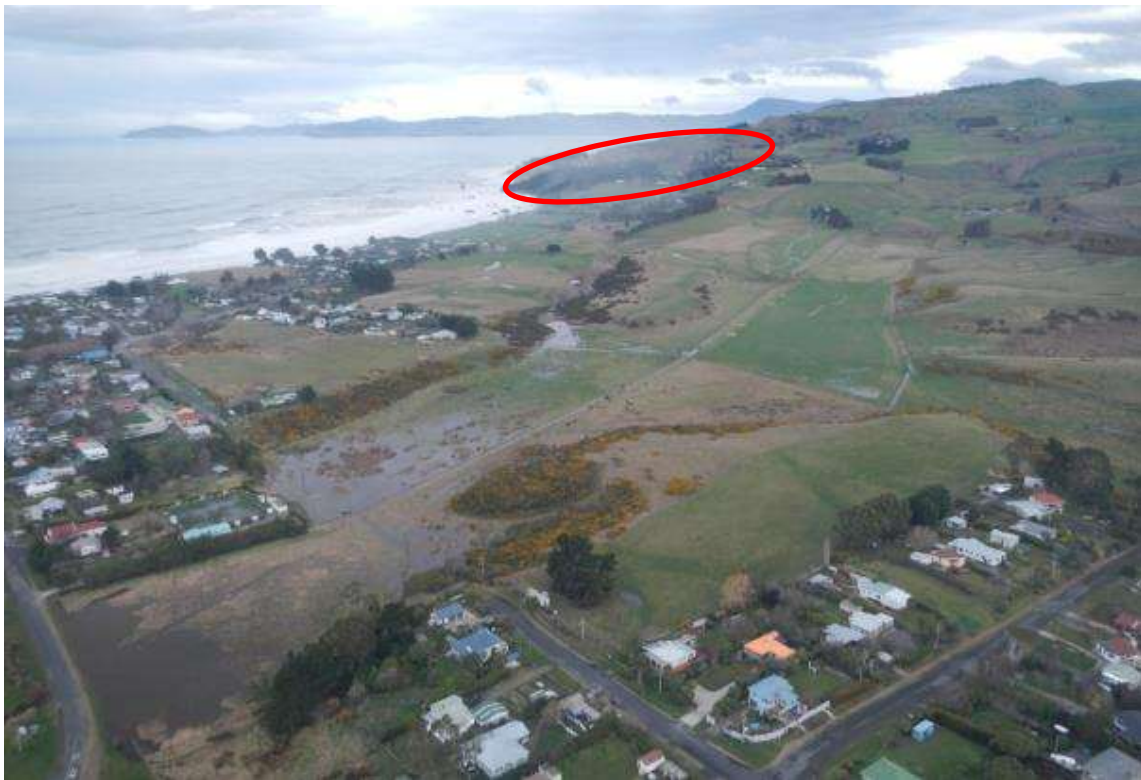
Figure 19 Aerial view towards the Puketeraki landslide from Karitane, following a period of heavy rainfall in August 2012. The red oval indicates the approximate location of the slide.
