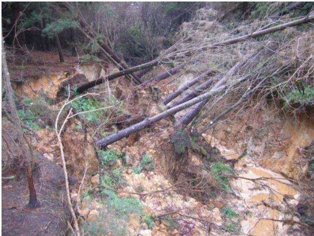
Figure 26 A view looking upstream showing the downstream limit of channel erosion in June 2008, caused in part by overflow of the pond. The pond is about 100 metres upstream from where this photograph was taken.
