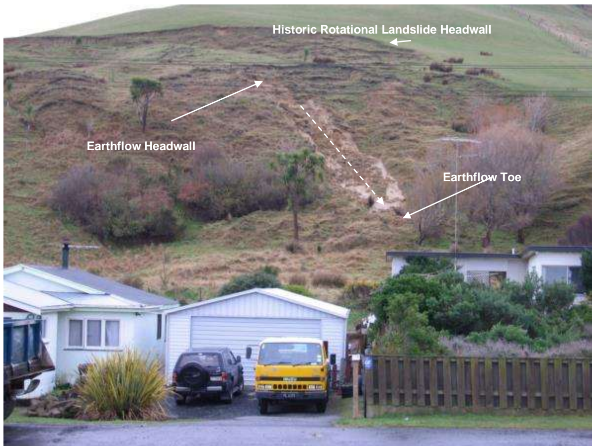
Figure 6 Evidence of recent movement on the Brighton Slide, 13 August 2008
