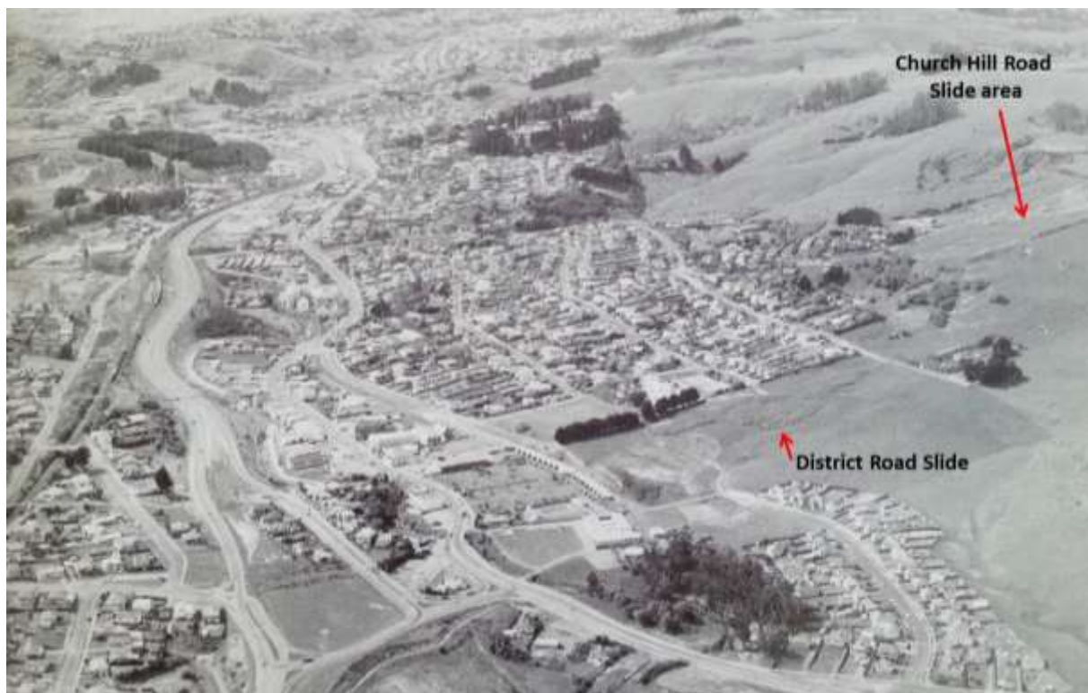
Figure 8 Oblique view east along Kaikorai Valley and Green Island, showing the District Road Slide and Church Hill Road Slide on the southern slopes. Background image from McKellar (1990), original date unknown
