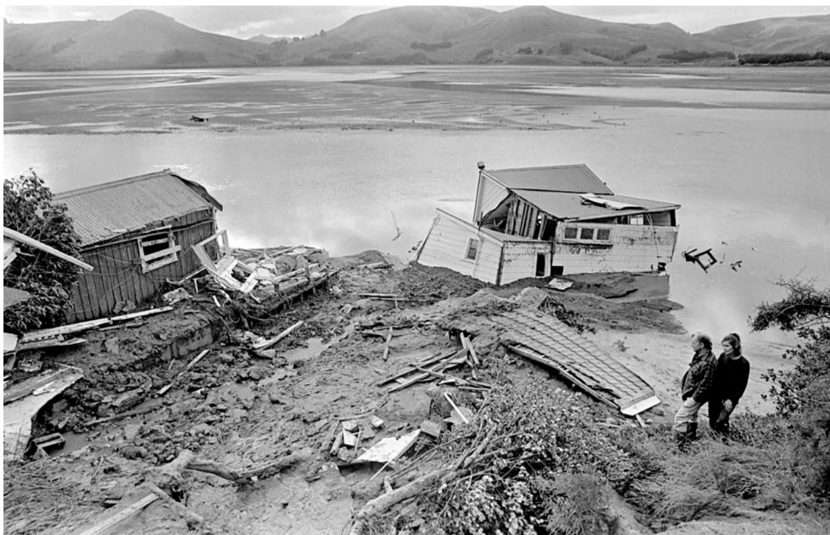
Figure 10 During the March 1994 rainstorm, a small landslide occurred in the head of a minor gully about halfway up Mt Charles, near Papanui Inlet, Otago Peninsula. The landslide material was mobilised into a debris flow that proceeded rapidly down the gully, crossed Cape Saunders Road and broke through the front gate of a holiday house built in the gully. Debris piled up against the house, which was broken off its foundations by the weight of debris and carried downhill several tens of metres before ending up in the Inlet, as seen in this view, looking north-northeast. The boatshed to the left largely escaped damage. The minor gully down which the debris flow came normally carried a small creek that ran past the house. This photo illustrates the potential hazard of landslide movement inundating a property, even though the landslide was initiated a long way from the property. Photograph courtesy of Otago Daily Times Newspaper, Jane Dawber, March 1994.
