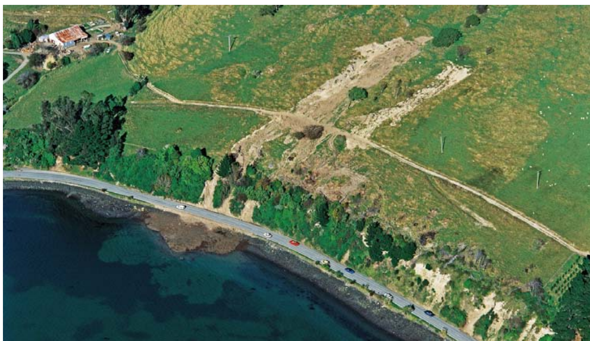
Figure 12 Surficial landslides occurred above Portobello Road, between Challis and Glenfalloch, during the March 1994 rainstorm, and generated debris flows that ran downslope, crossed the road and accumulated in Otago Harbour. The photo was taken after the debris had been cleared off the road, although the debris remains evident on the foreshore (brown) and seabed (pale). Being one of only two access roads to Otago Peninsula, this photo illustrates the potential vulnerability of this key transport route for peninsula residents. Photo: GNS Science, D.L. Homer, CN32057b, 1 May 1994.
