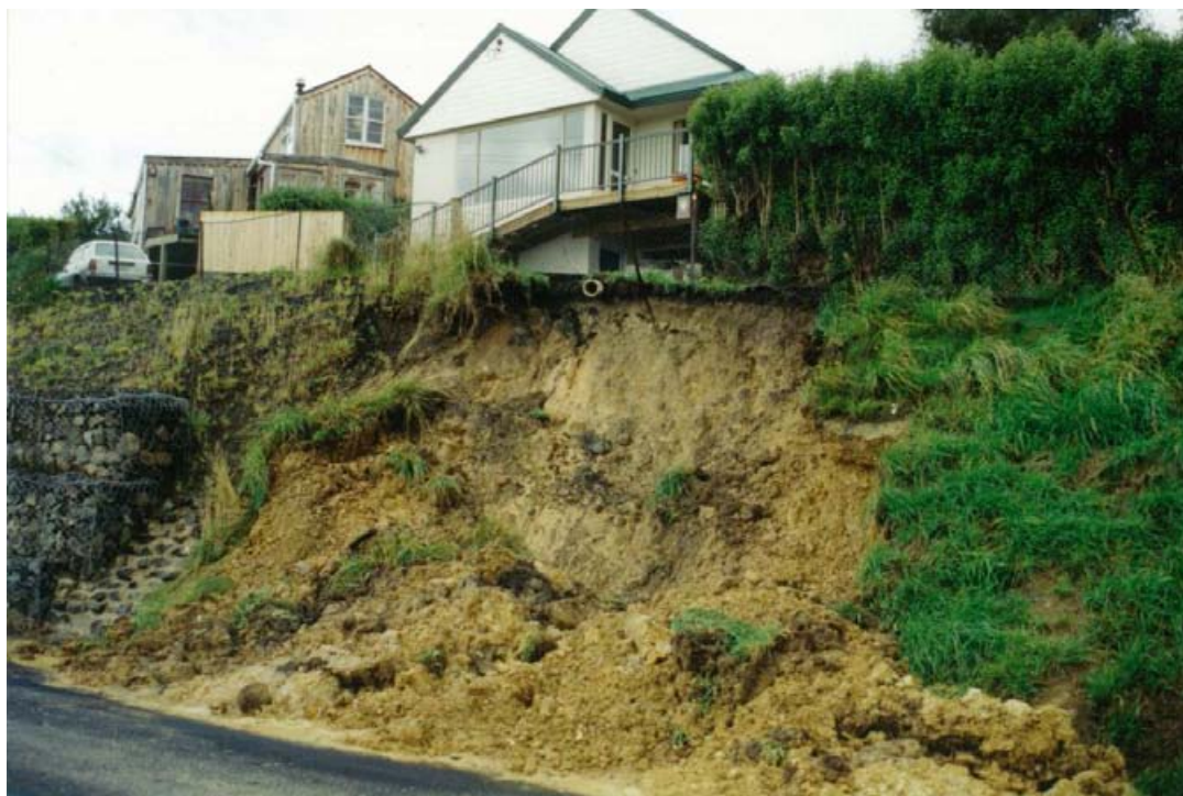
Figure 11 A small surficial landslide from this road cut in Margate Ave, Broad Bay, resulted from the March 1994 rainstorm. Flow from the drain at the head of the slide may have contributed to the failure. However, the gabion wall to the left indicates that this slope has previously experienced instability, which the gabions were doubtless installed to remediate. This photo illustrates the potential hazard of landslide movement undermining a property. Photo: GNS Science, I.M. Turnbull, 20 March 1994.
