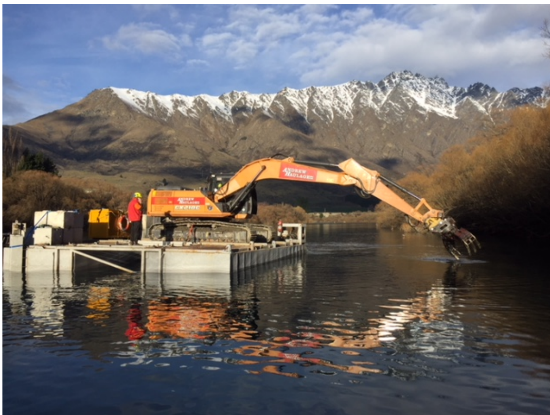
The barge and excavator working in the Kawarau River to remove submerged willows
