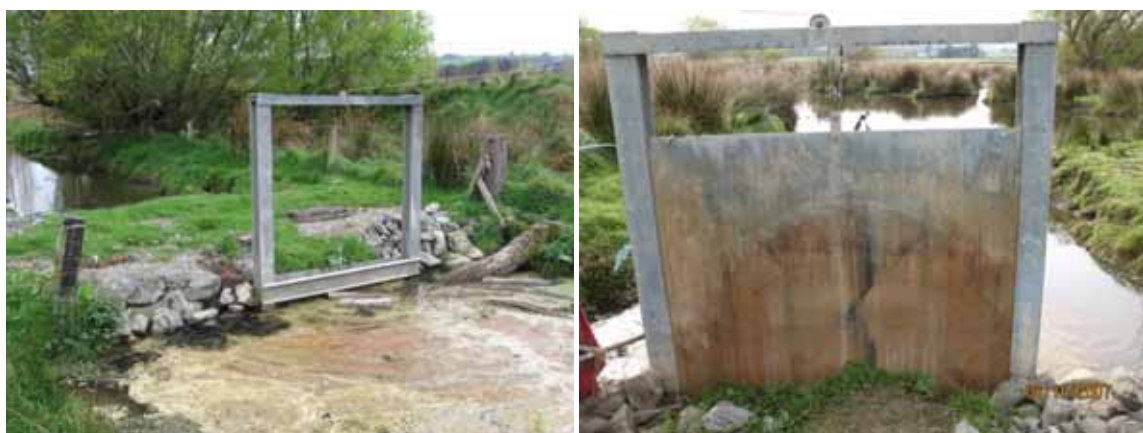
Figure 7 The diversion drain control gate (shut and open).
