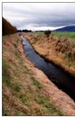
Site 18 Main Drain @ Miller Rd
