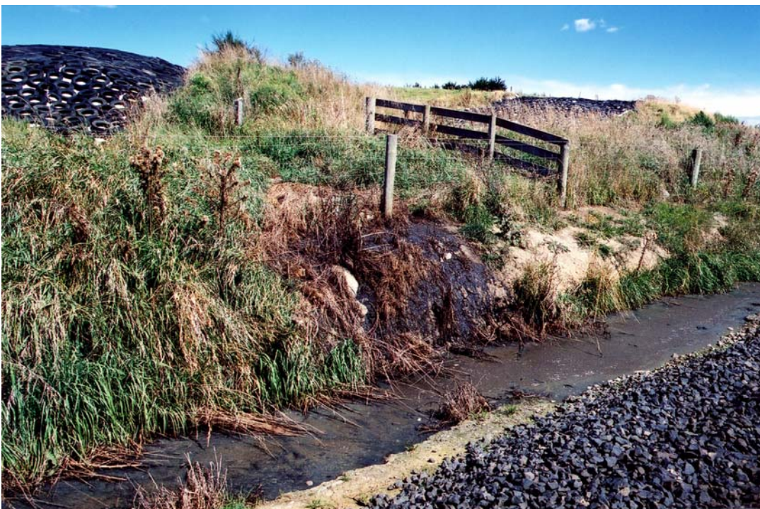
Figure 5.12 Leachate runoff from a silage pit below Riverside Road, near Owhiro Stream
