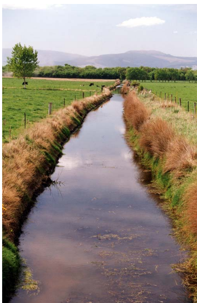
Figure 5.13 The A1 Drain upstream of Riverside Road. The drain is fenced off preventing stock access and riparian vegetation has been allowed to grow
