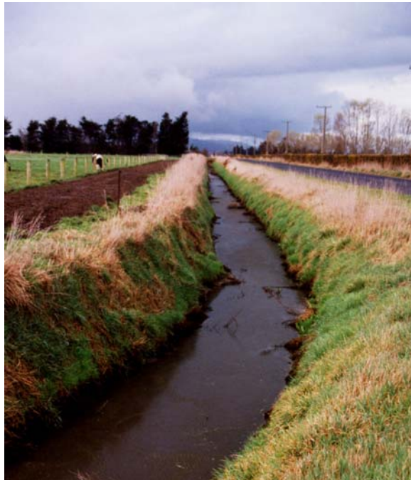
Figure 3.13 Kirks Drain at Marshall Road
