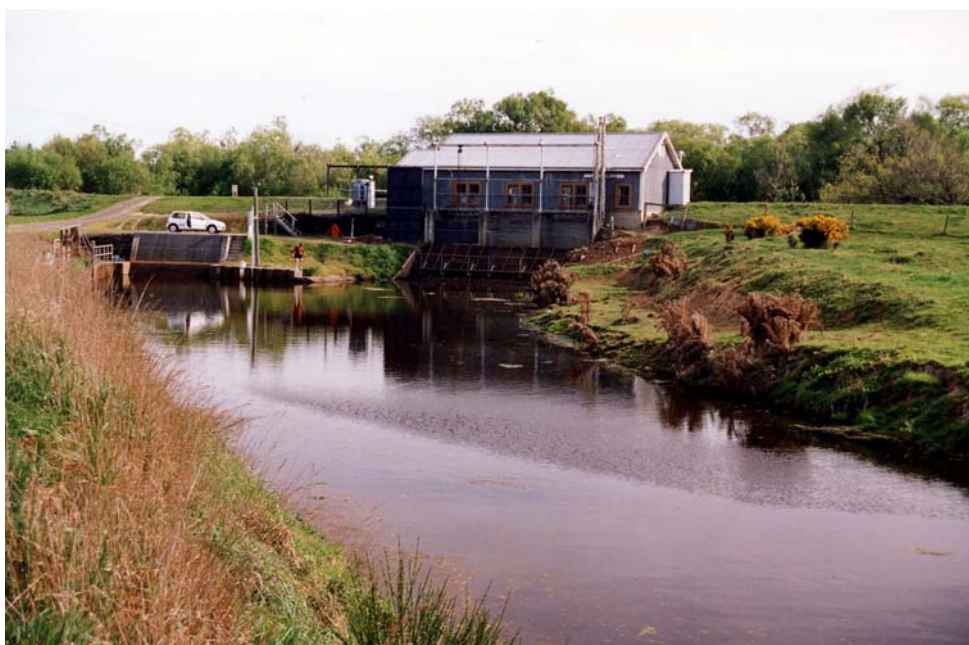
Figure 3.12 Taieri Main Drain at the Waipori Pumping Station
