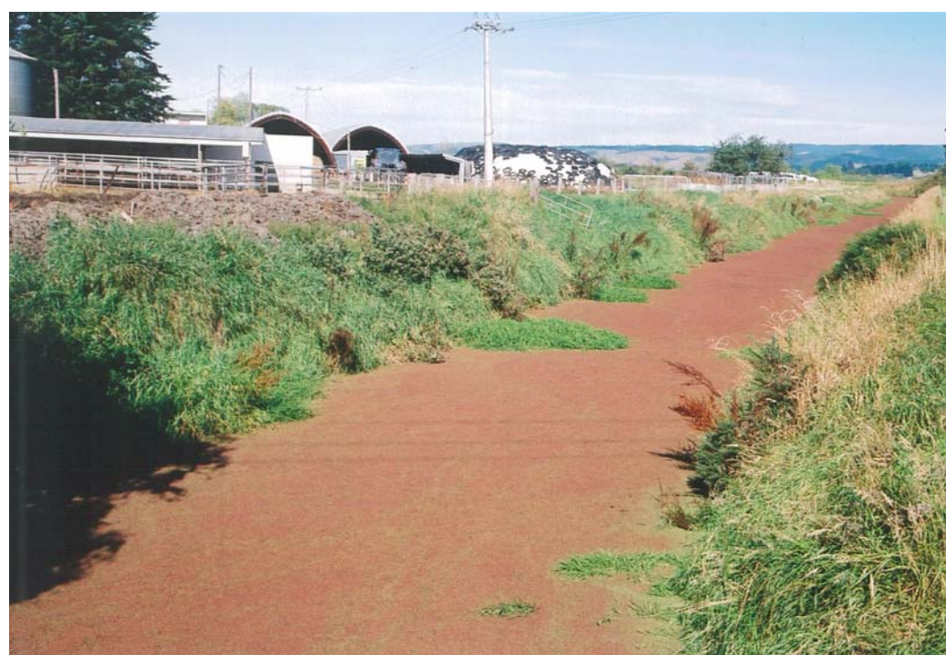
Figure 5.10 The Main Drain at Marshall Road looking downstream in September 2001 (top) and in March 2002 (bottom) when the drain was smothered with Azolla
