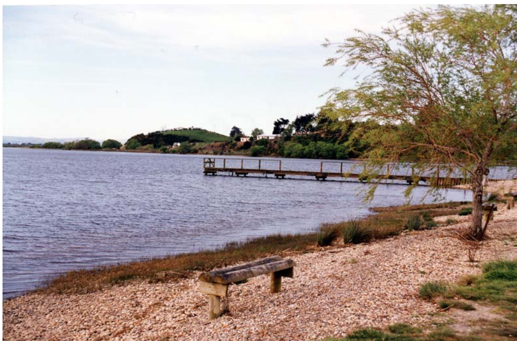
Figure 3.15 Boat jetty at Lake Waihola
