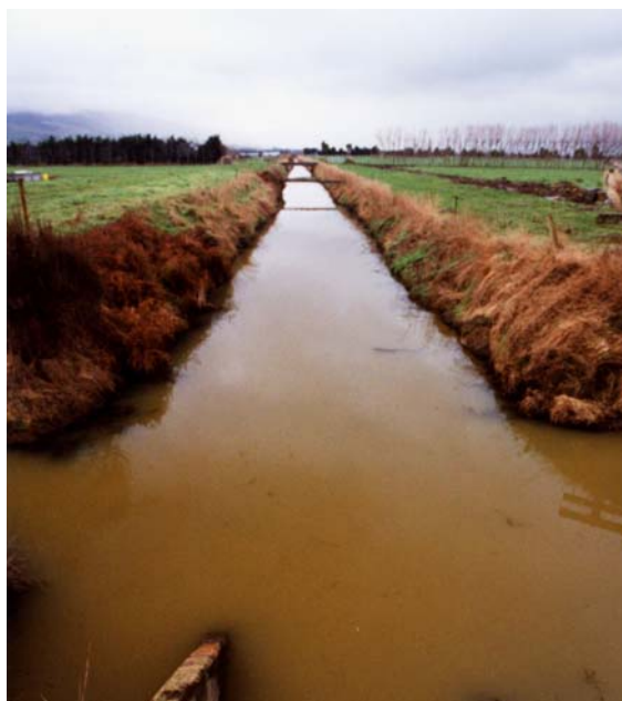
Figure 3.14 Lee Canal Drain at Marshall Road
