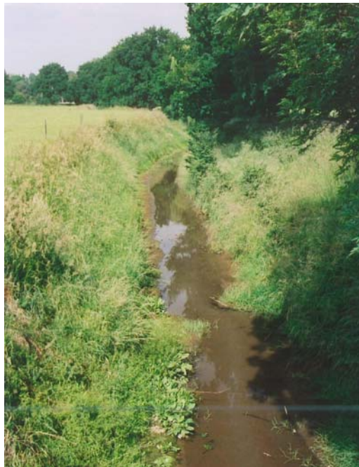
Figure 3.11 O13 Drain looking downstream from Riverside Road
