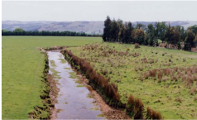
Figure 3.10 A1 Drain from the Taieri River flood gates
