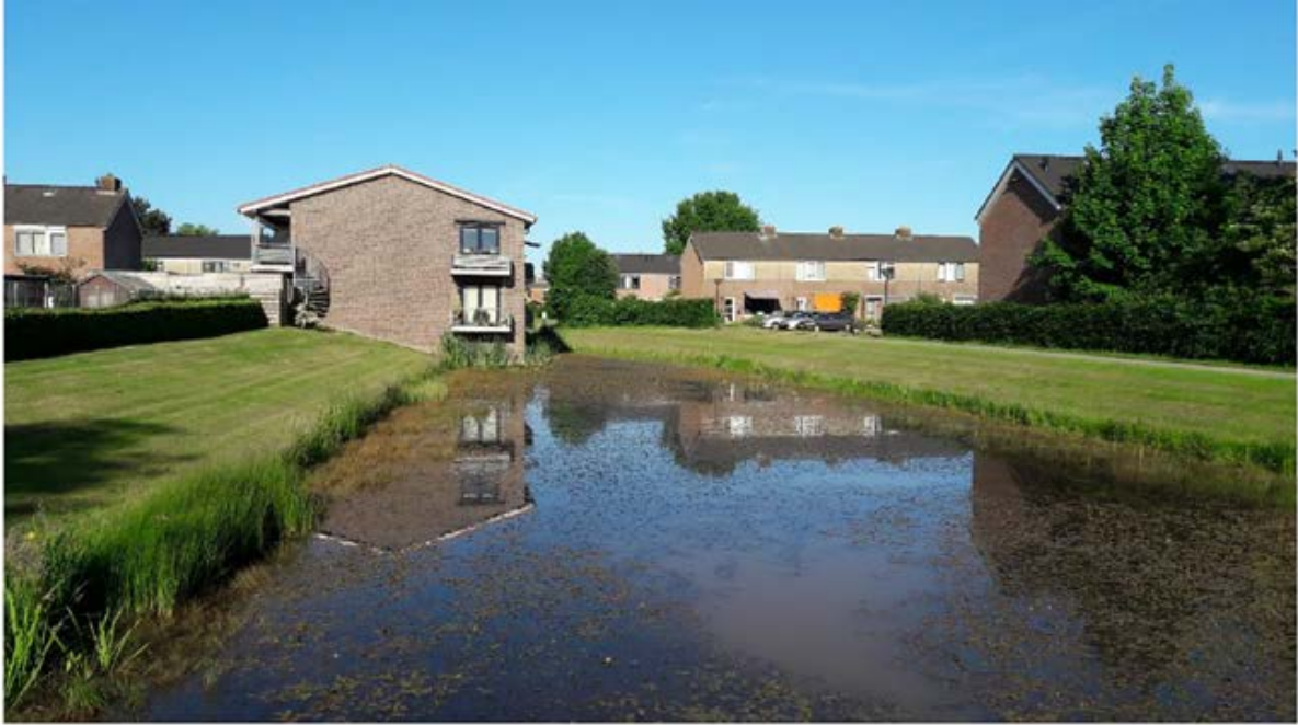
Figure 3: Greater New open canal dug during the district renovation of Oosterwolde-Zuid: water storage, drainage, improved water quality and overall quality of the public space.
