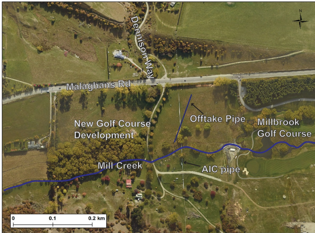
Figure 7. Location of the offtake pipe at Millbrook’s Dalgleish Farm development. The Arrow Irrigation Company pipe visible in photo has since been re-routed. Mill Creek will eventually be diverted (by Millbrook) to the north.
