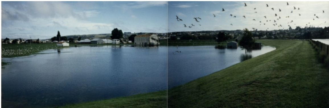
Figure 4.18 Localised ponding due to seepage coming from the relief wells on the landward side of the floodbank at the Balclutha Showgrounds during the March 1987 flood event (2300 m 3 /s at Balclutha).
