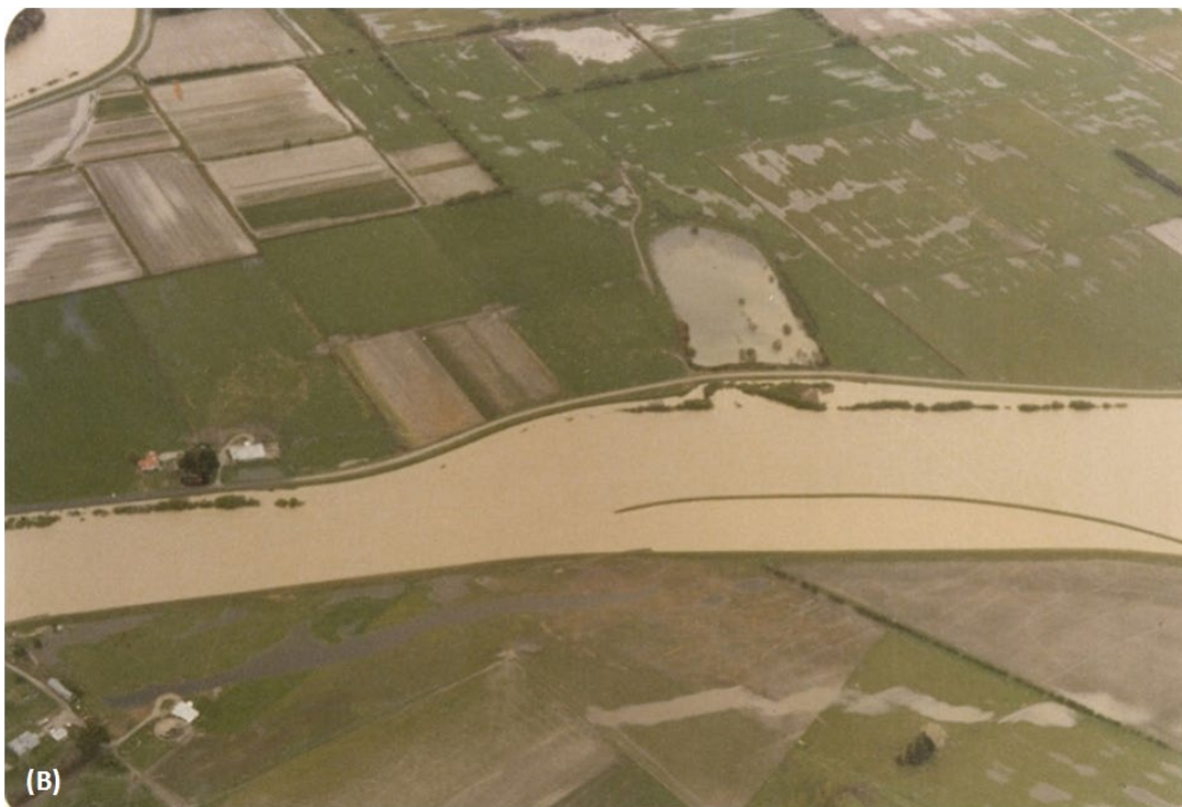
Figure 4.25 Location of Weirs Gap (A) and Weirs Gap during the October 1978 flood event (B). Note the water from seepage under the floodbank ponding on the landward side of the floodbank in the balancing pond.
