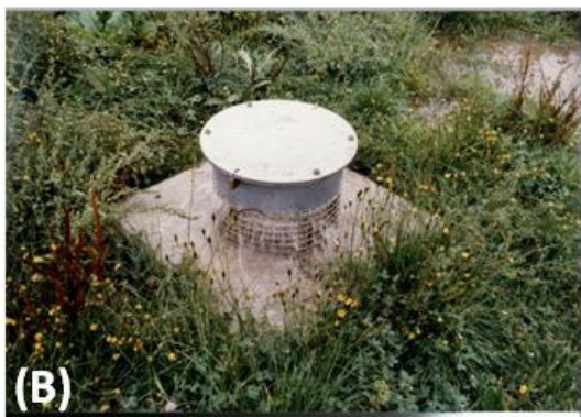
Figure 4.7 Location of the 43 relief wells in Balclutha a) and photos of the emerging part of two types of relief wells operating in the March 1987 flood event ( b and c , below).
