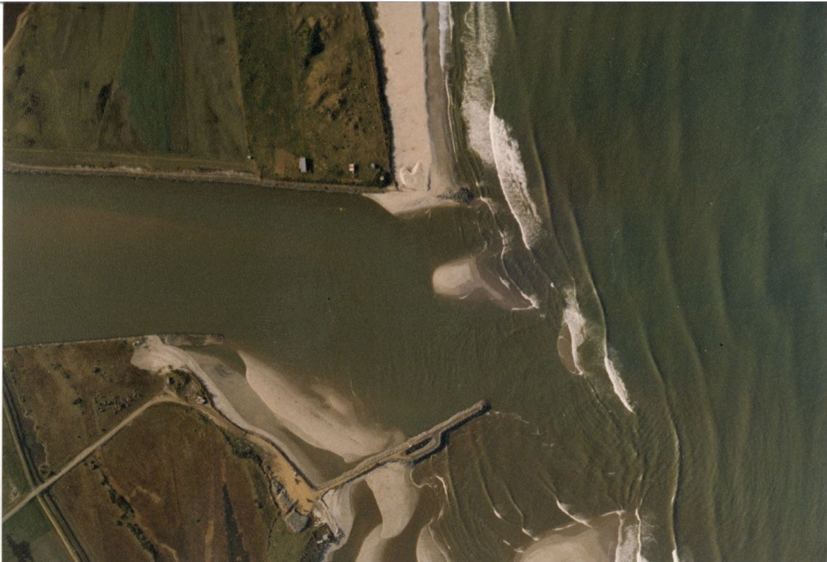
Figure 4.4 Koau Mouth works- June 1983 (during construction).
