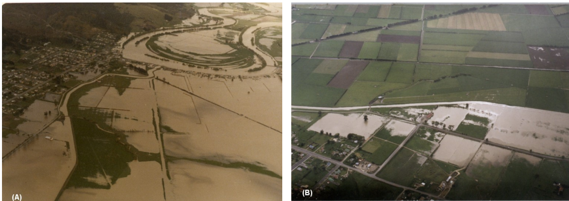
Figure 4.39 Area 22 during (A) the October 1978 flood, with Area 22 to the left foreground; (B) the November 1999 flood. The photos were not necessarily taken at the peak of those flood events.
