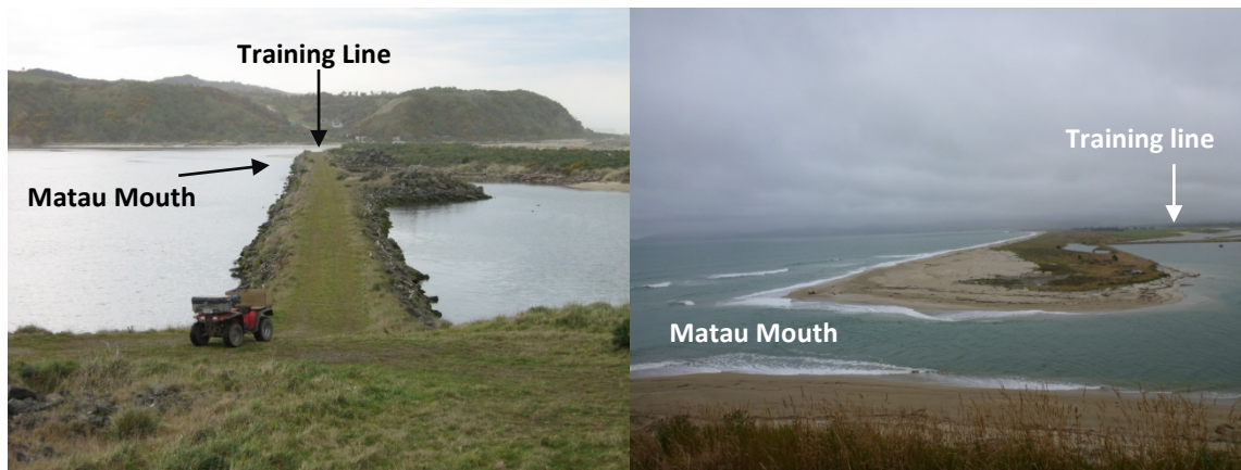
Figure 3.13 Training line on the true right of the Matau Mouth of the Clutha River/Mata-au. Left image is looking eastwards, towards the Matau Mouth (September 2006), right image is looking westward towards Molyneux Bay (March 2013).
