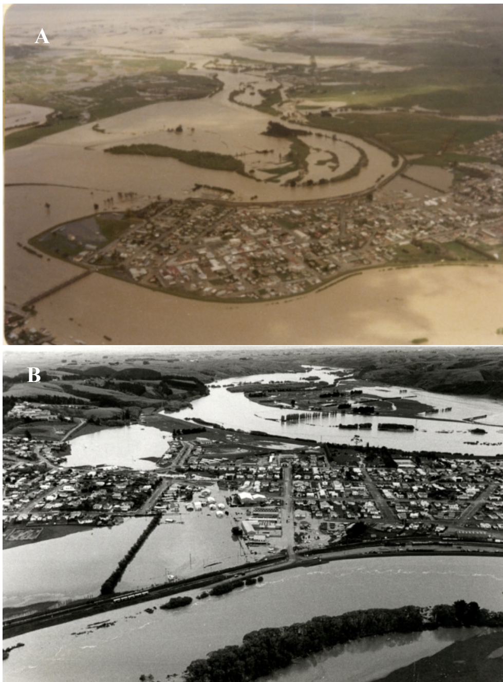
Figure 4.22 Flooding in Balclutha during the October 1978 flood event (estimated peak flow of 4580 m 3 /s at Balclutha) (a) looking south. Note ponding behind the floodbank within Area 3. (b) Looking north. Note ponding from Hospital Creek and/or rainfall accumulation (not shown in a).
