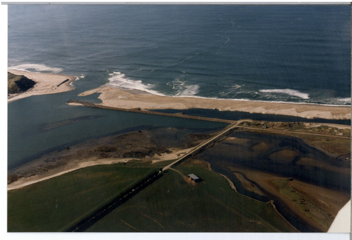
Figure 4.5 Matau Mouth works - September 1993
