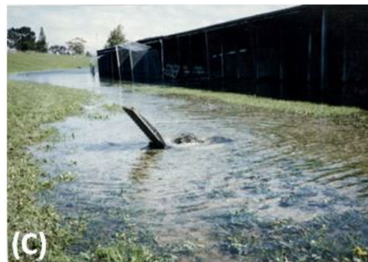
Figure 4.7 Location of the 43 relief wells in Balclutha a) and photos of the emerging part of two types of relief wells operating in the March 1987 flood event ( b and c , below).
