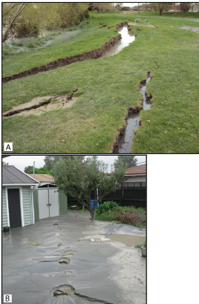
Figure 5.3 a) Lateral spreading on the true-left bank of the Kaiapoi River, after the Christchurch magnitude 6.3 earthquake. b) Sand boils in Avonside after the Christchurch earthquake in February 2011 (after Quigley et al. , 2013).
