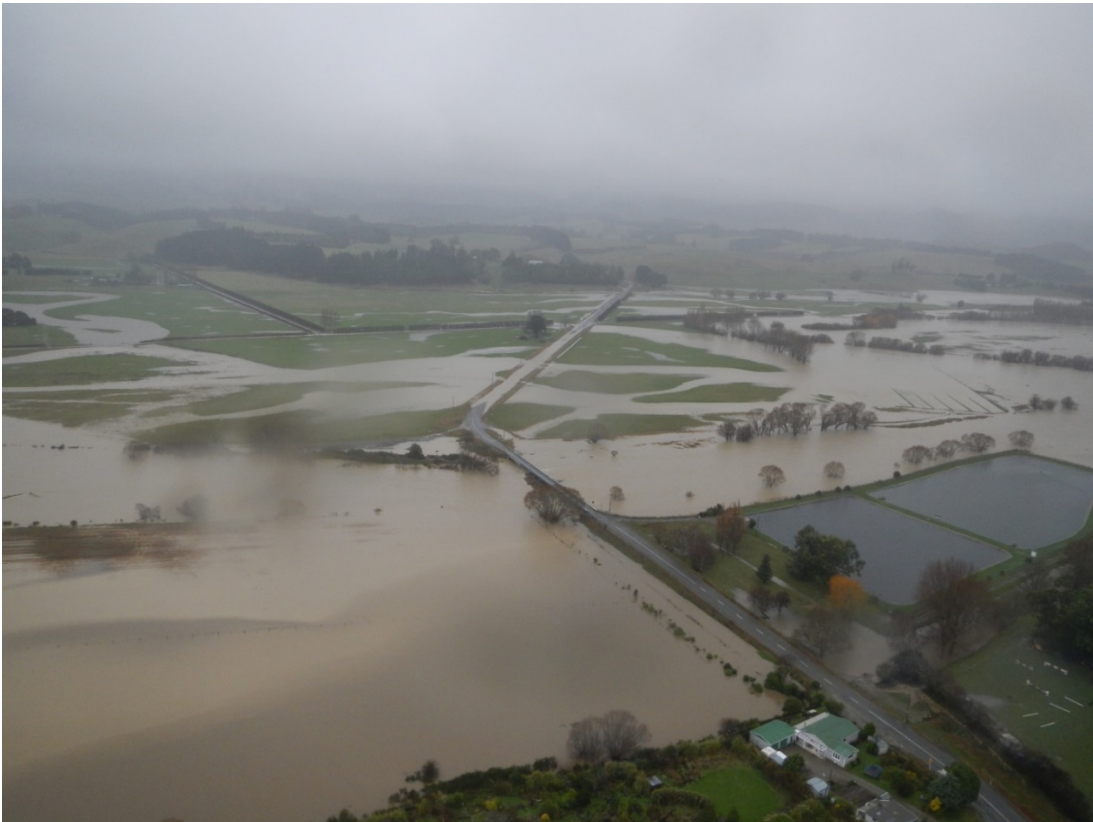
Figure 9. Shag River/Waihemo in flood, looking downstream at the Horse Range Road bridge (June 17, 2013)
