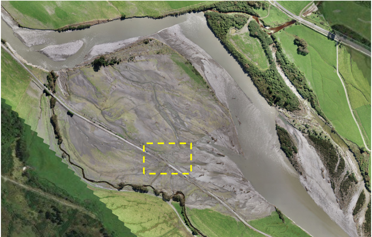
Figure 1. Drone photo showing damages to the Arahura Valley Road (centre) and debris deposition caused by overtopping of the Arahura River banks. See next figure for close-up (yellow rectangle) – March 2019 (source: West Coast Regional Council).
