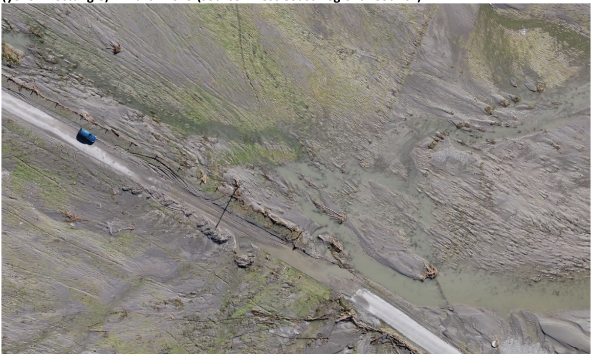
Figure 2. Close-up from drone photo showing damages to the Arahura Valley Road (centre) and debris deposition caused by overtopping of the Arahura River banks – March 2019 (source: West Coast Regional Council)
