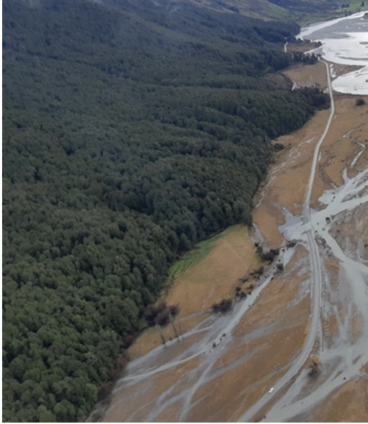
Figure 6: Top: Channel position – 2007 (left) and 2019 post March 2019 high flows (right) Bottom: Kinloch Road flooding between Turner Creek and Glacier Burn – 31 May 2019
