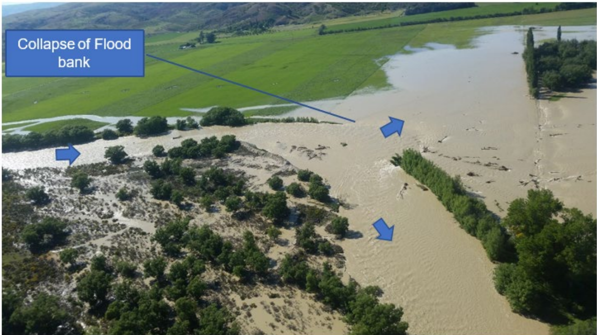
Figure 8: Manuherikia River – Left bank overflow – November 2018
