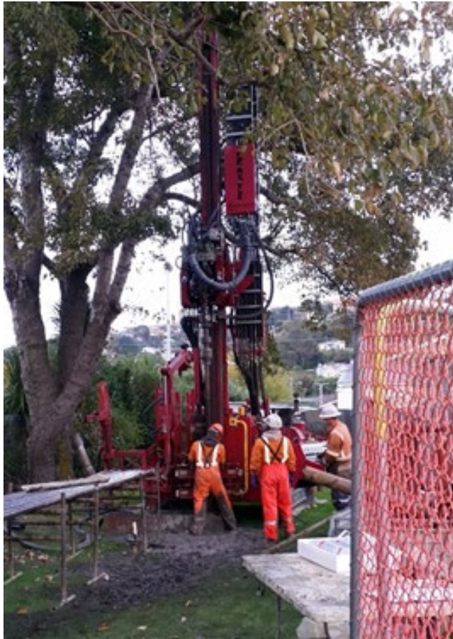
Figure 1: Drilling to bedrock at Tonga Park (NZSR01), South Dunedin 22 May 2019.
