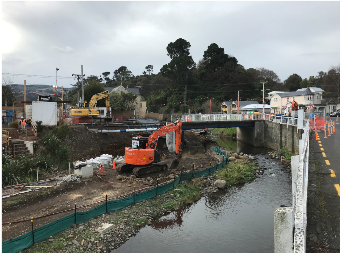
Figure 2 Dundas St Bridge stage of the Leith Flood Protection Scheme
