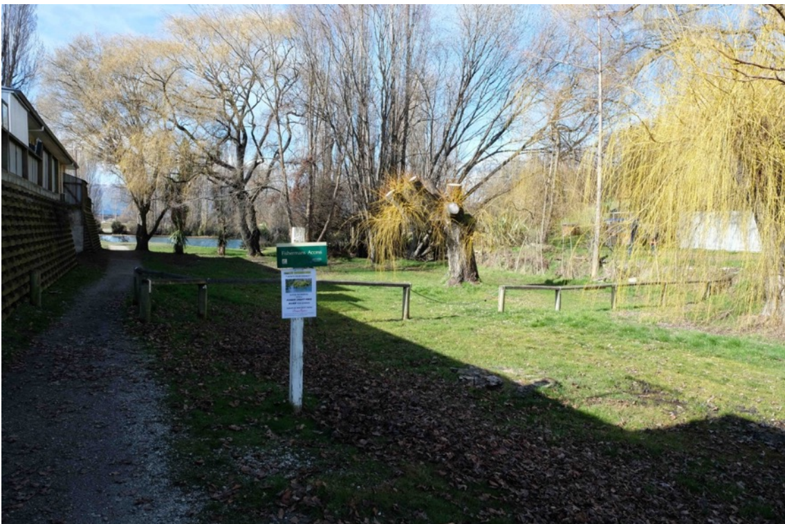
Figure 31 Reserve between Pump Station 12 and the Clutha River.
