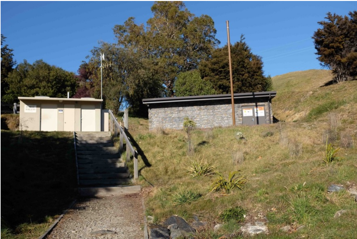
Figure 62 Pump Station 33 on Scotts Beach Road on the shore of Lake Hāwea.
