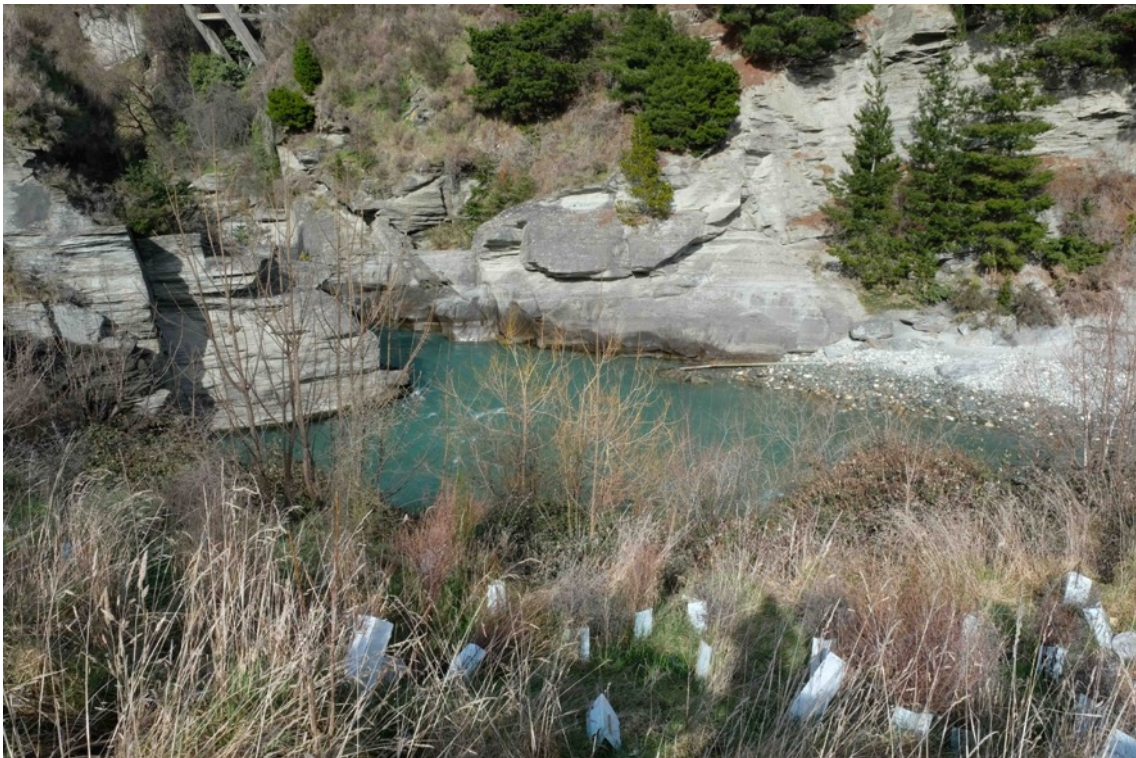
Figure 46 View towards Pump Station 22 (Oxenbridge Tunnel Road) from the opposite (true left) bank of the Shotover River.
