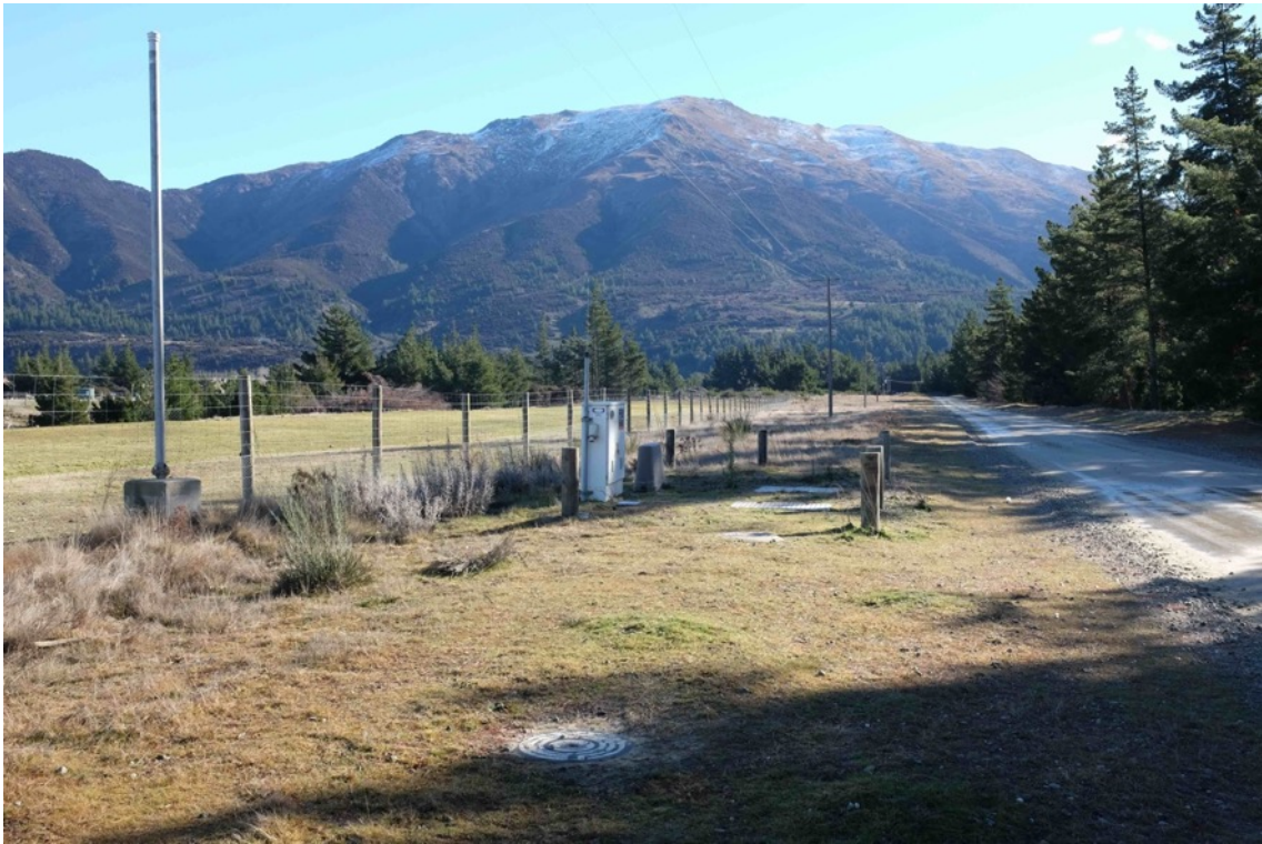
Figure 64 Pump Station 34 on Domain Road near Lake Hāwea.
