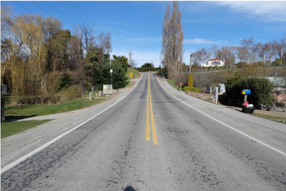
Figure 30 Pump station 12 on Alison Avenue, Albert Town.
