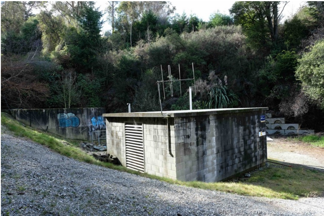
Figure 50 Pump Station 24 near Glenorchy-Queenstown Road.
