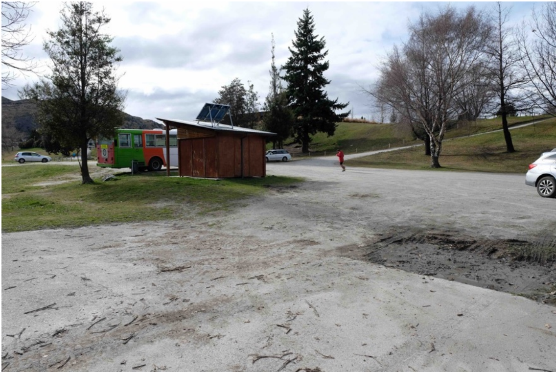
Figure 54 Area of sewer main with overflow on lake shore of Lake Wakatipu at Frankton Beach on Allan Crescent.
