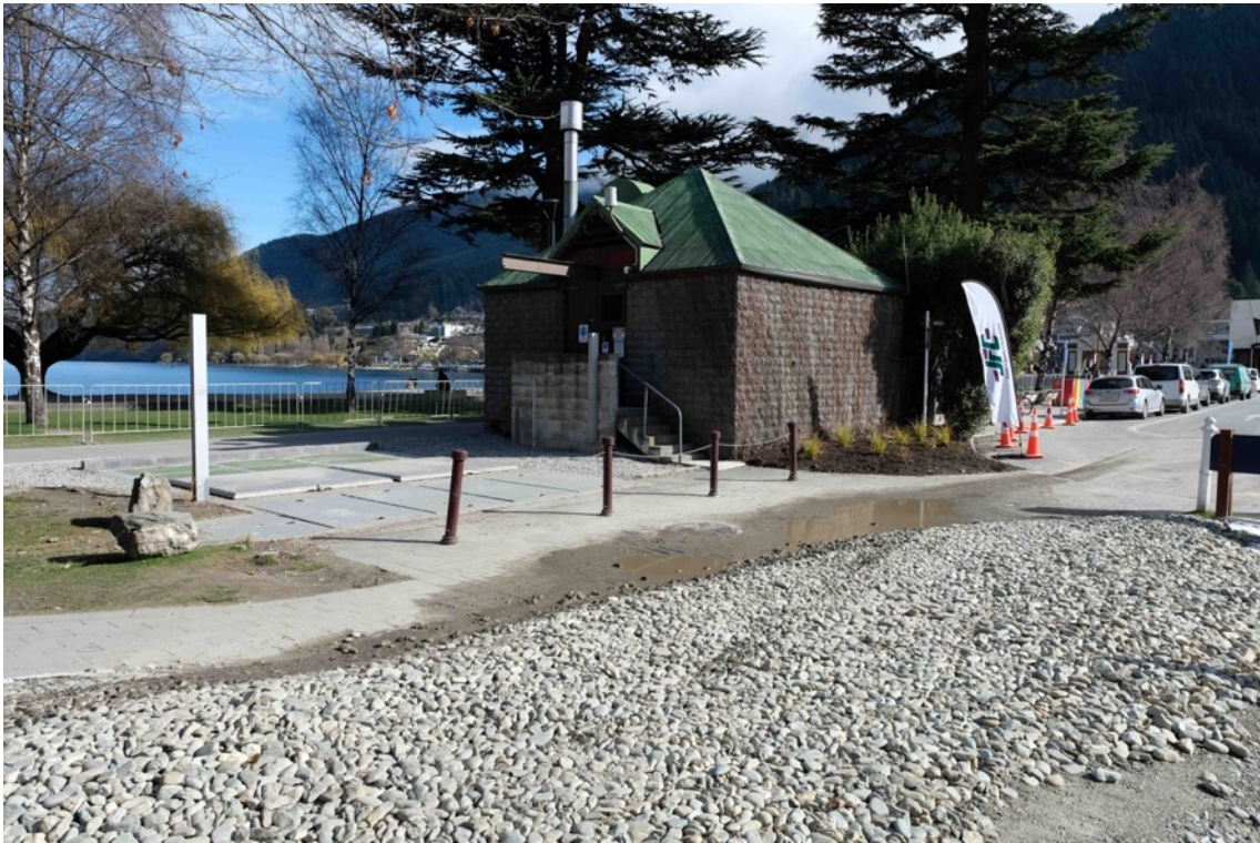
Figure 47 Pump Station 23 on Marine Parade on the shore of Queenstown Bay, Lake Wakatipu.
