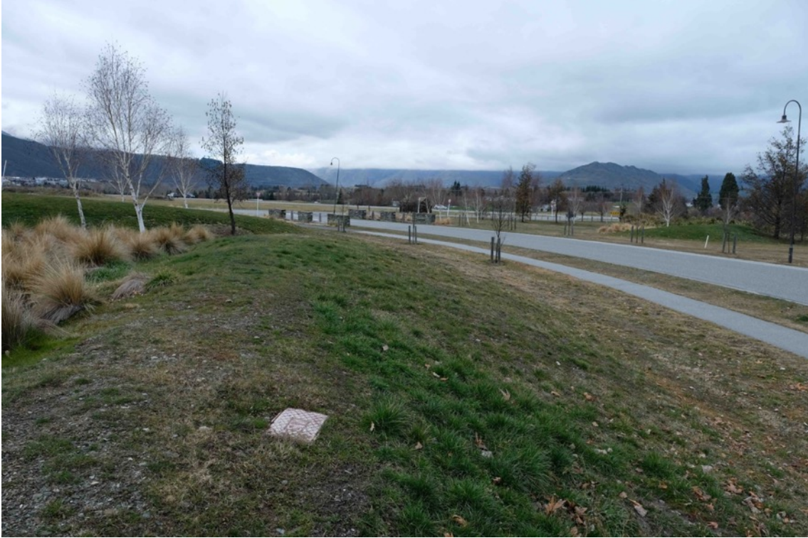
Figure 43 Pump station 20 beside Essex Avenue, Arrow Town.
