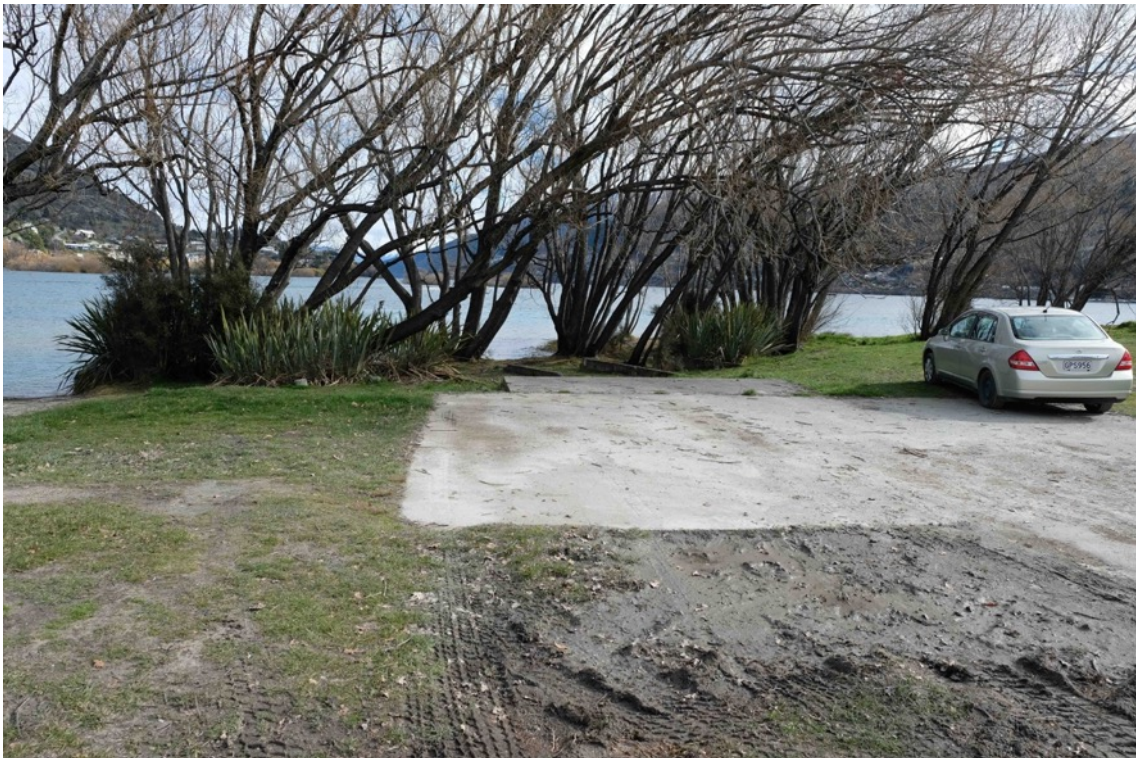
Figure 55 Area of sewer main with overflow on lake shore of Lake Wakatipu at Frankton Beach on Allan Crescent.
