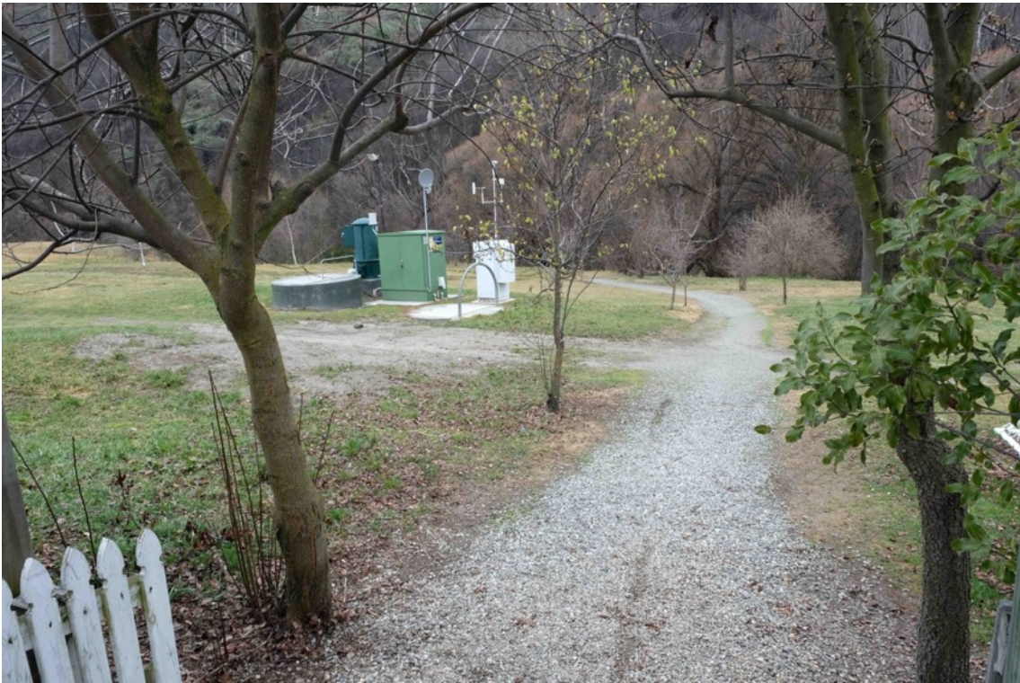
Figure 37 Pump Station 18 near Alexander Place, Arrow Town.
