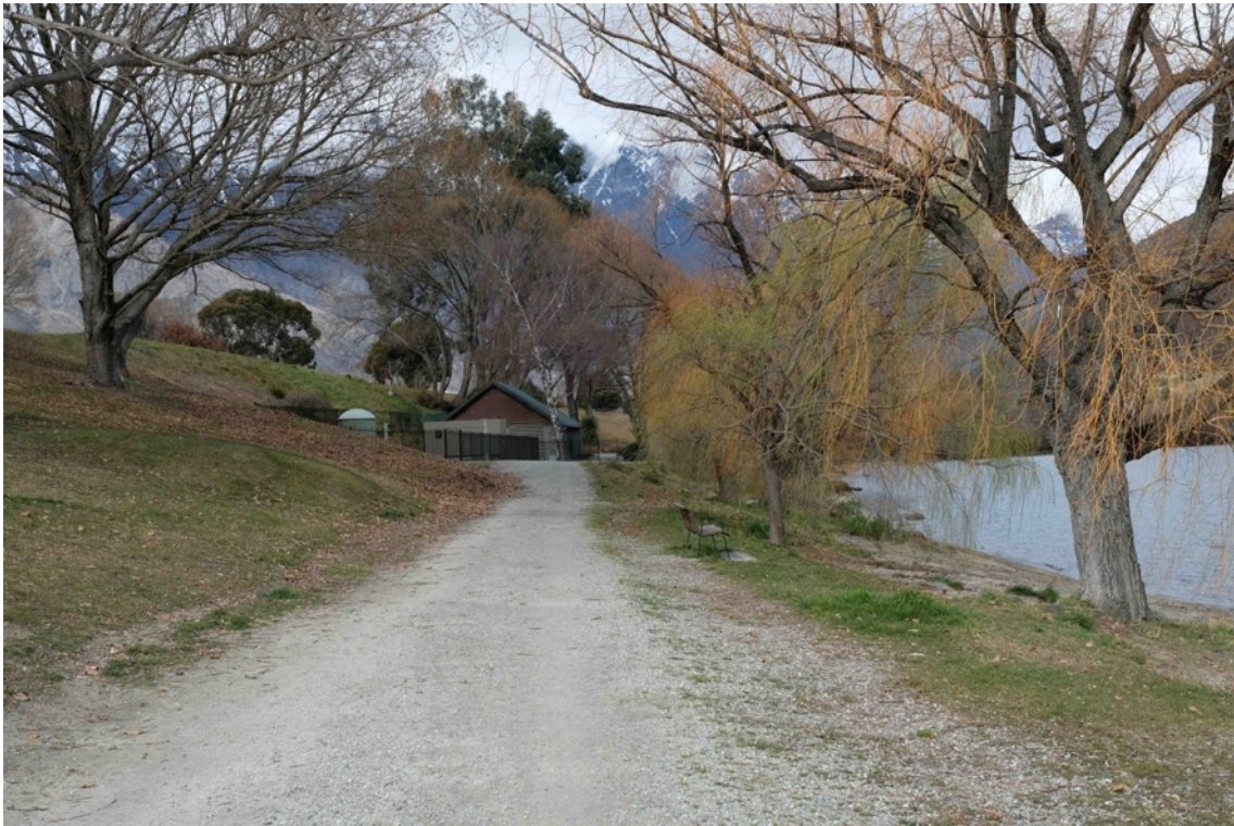
Figure 52 Pump Station 25 on the shore of Lake Wakatipu at Frankton Beach.
