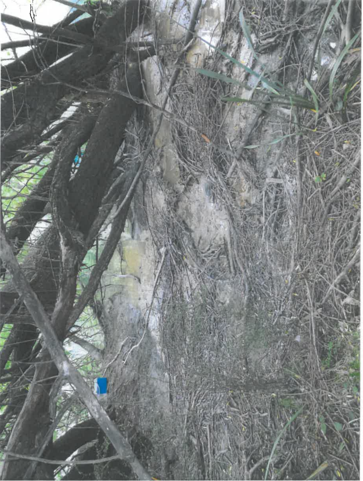
View looking at the downstream end of the sewage flow where it entered the river.
