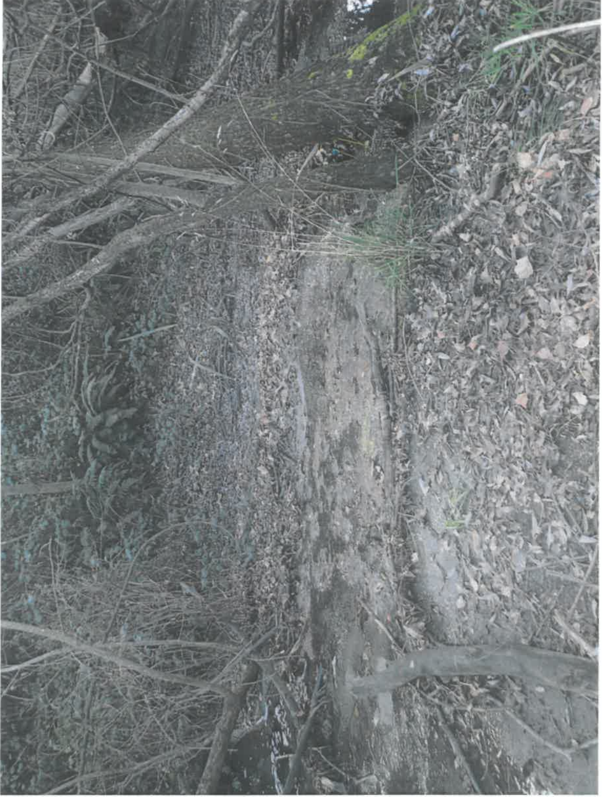
View looking back towards but to right of stormwater pipe outlet.
