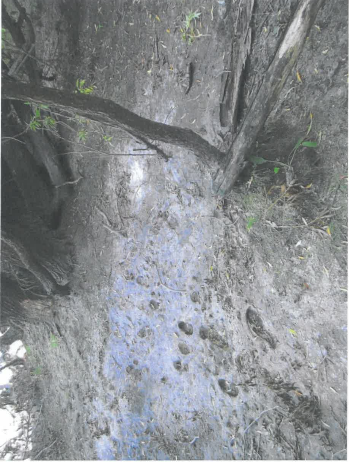
View of ponded area and sewage flow path. Note: foot prints in sewage sludge.
