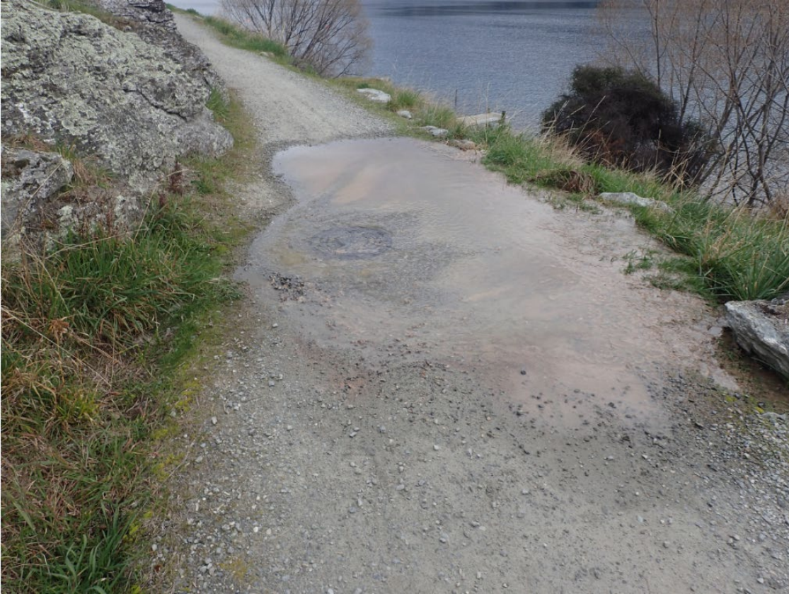
Photograph 3 Discharge overflowing from a manhole across the Kelvin Heights public track adjacent to Loop Road, before flowing into Lake Wakatipu 3 .
