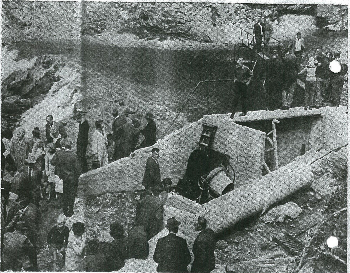
KEY to the Criffel irrigation scheme is this dam on the main branch of the Luggate Creek. Because of fluctuations in the level of the creek it was necessary to ensure an even supply of water for the outlet pipeline (lower right). The catwalk extending out over the dam gives access to a gate which can open and close the safety valve pipe built into the face of the dam.
