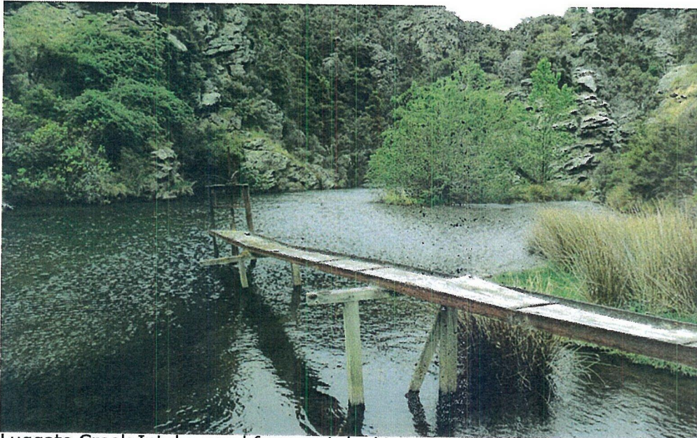
Luggate Creek Intake pond from weir looking south upstream. Shows walkway and gate control for 900 diam discharge pipe through weir
