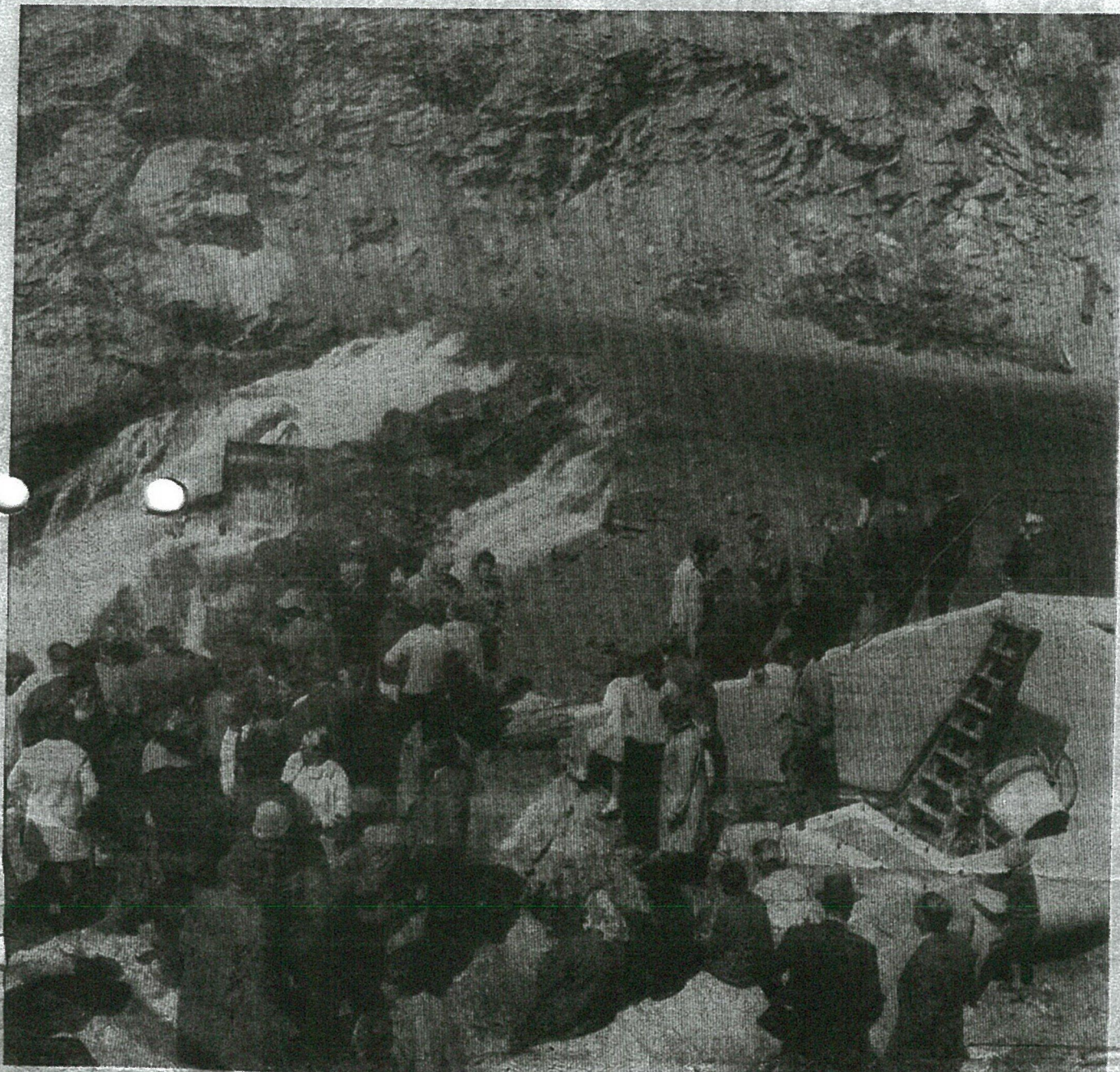
PRIVATE IRRIGATION SCHEME. —Some of the many visitors to the Criffel station on Saturday inspecting the weir built across the Luggate Creek. When completed, the scheme will eventually irrigate 2,000 acres, and was built and financed by four farmers in the Mt. Barker region.
