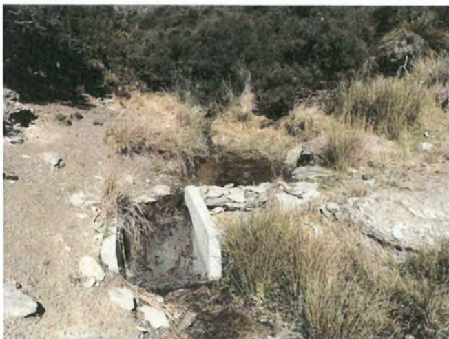
Water is being abstracted under Permit 97803 at this location (trib of Aliceburn) E1301861 N5033204. Screen in place and junction box / break tank.
