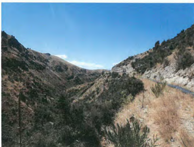
2008.519 & 97803 Aliceburn River, main pipeline to overflow tank.
