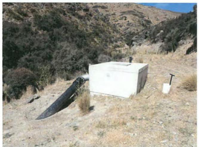
Water is being abstracted under Permit 97803 at this location (trib of Aliceburn) E1301861 N5033204. Screen in place and junction box / break tank.
