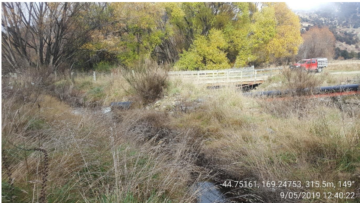
Figure 2: LIC pipe taking Alice burn water over the Luggate and combining it with the LIC Luggate Creek race.
