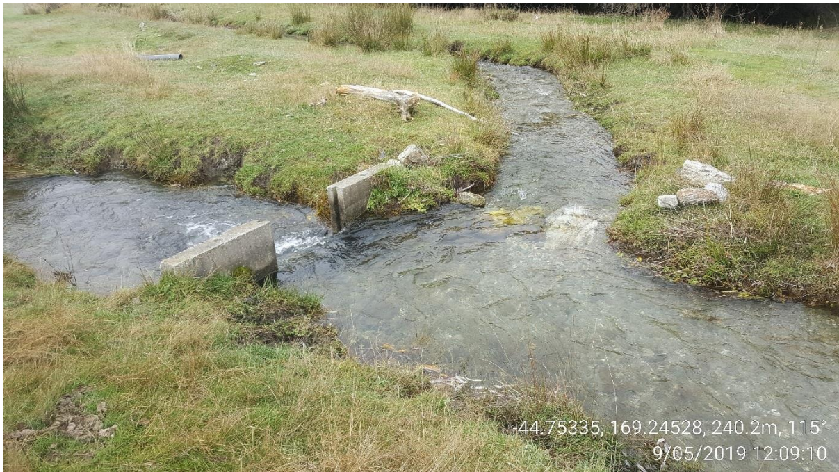
Figure 3: LIC race taking water from the Alice Burn. The Alice burn take is ~10m upstream of this point in the race. A bywash provides an opportunity for the water to return to the Alice Burn before the confluence with the Luggate mainstem.
