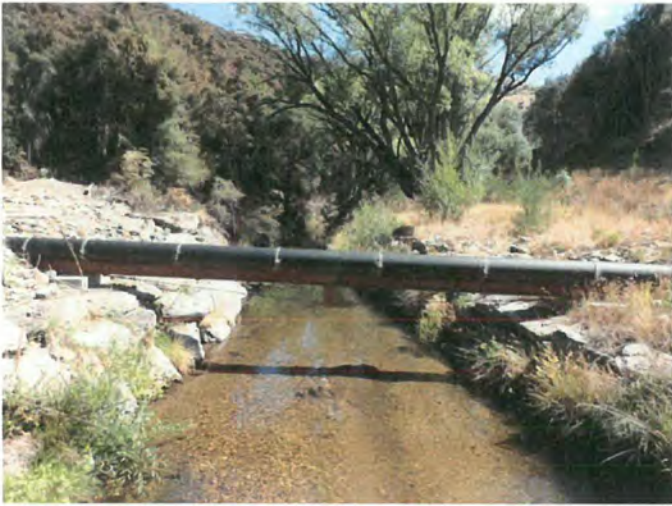
Race for WR7285cr & WR7298cr, a tributary of Luggate Creek – race enters pipe over Luggate Creek to join take from Luggate Creek.
