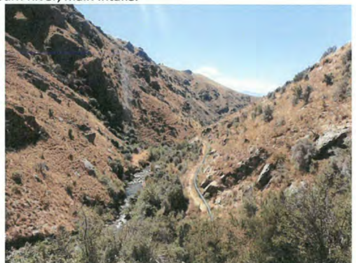
2008.519 & 97803 Aliceburn River, main pipeline to overflow tank.
