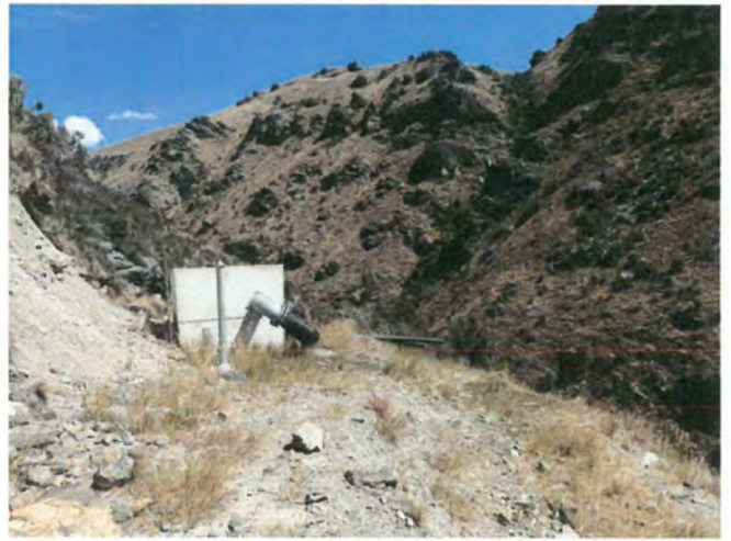
2008.519 & 97803 Aliceburn River overflow tank – overflow goes back in to the Aliceburn River. Overflow located at E1300519 N5032996.
