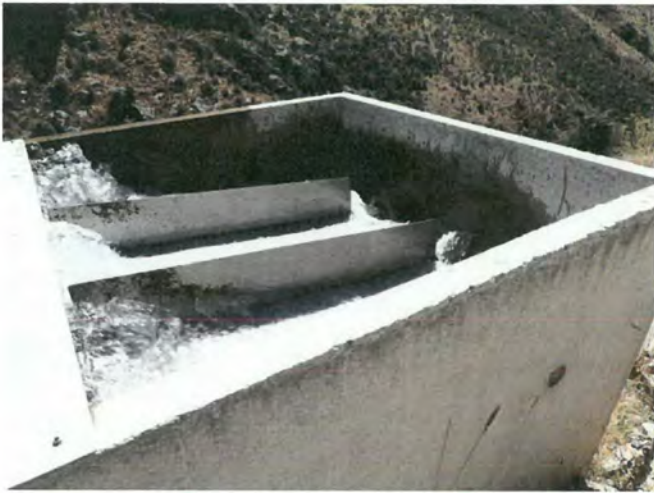
2008.519 & 97803 Aliceburn River overflow tank – overflow goes back in to the Aliceburn River. Overflow located at E1300519 N5032996.
