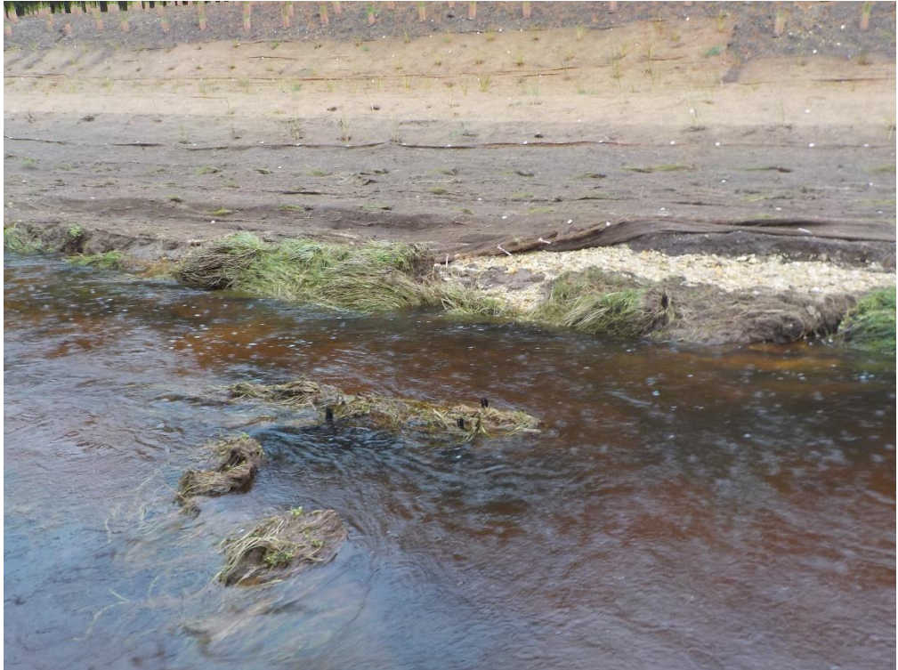
Figure 1: Waituna Creek with replanted stream banks and log cover in the stream channel
