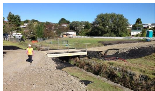
Figure 113: A temporary bridge in the process of being installed
