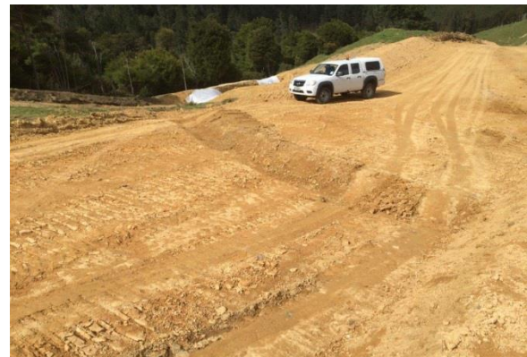
Figure 22: Contour drain installed across access track
