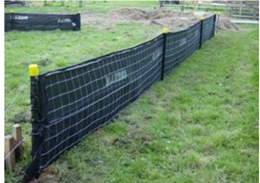
Figure 86: Super silt fence
