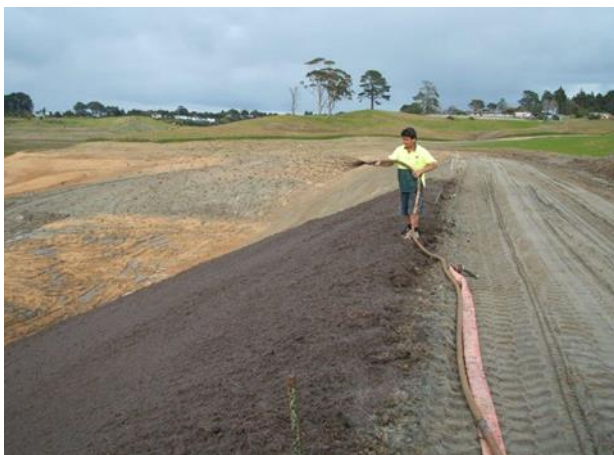
Figure 54: Hydromulch application
