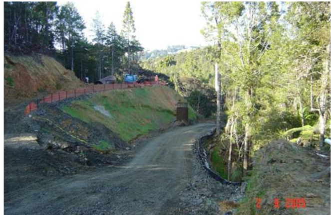
Figure 10: Northern Motorway construction site - minimising disturbance
