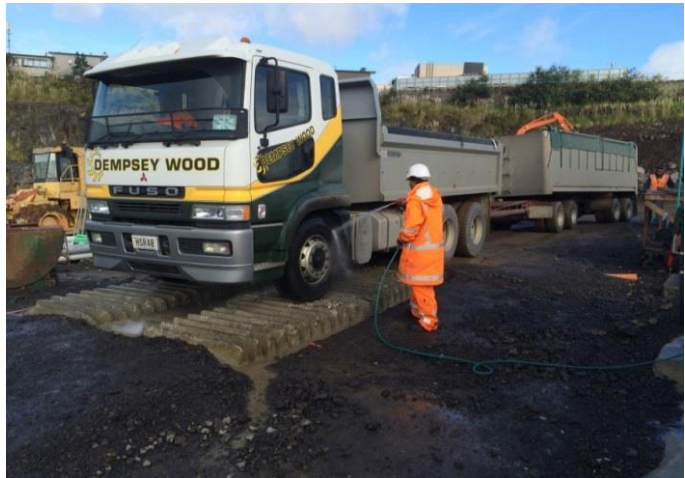
Figure 36: Example of truck wash and shaker ramp
