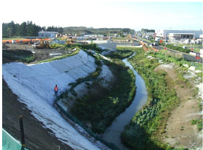
Figure 57: Geotextile used to temporarily stabilise the batter face
