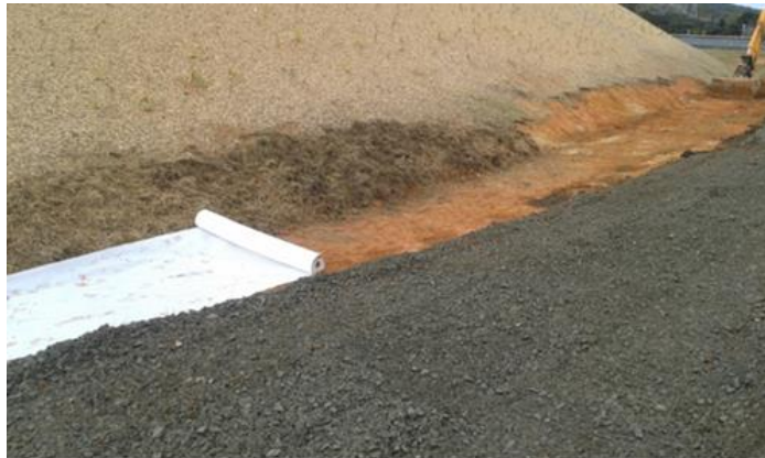
Figure 41: Stabilisation via a combination of chip mulch, geotextile and aggregate
