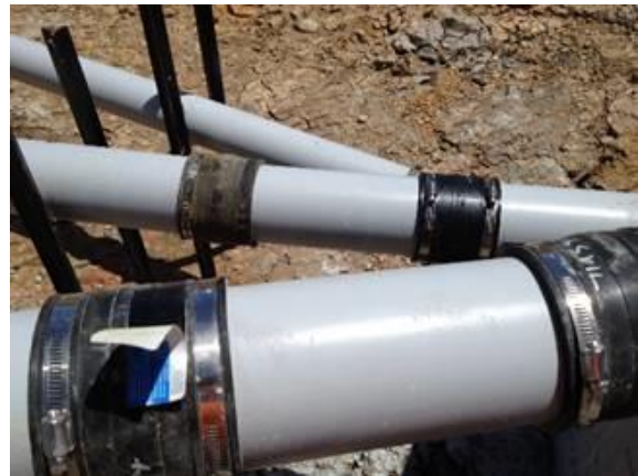
Figure 76: Steel strapping used to attach decant system to horizontal pipework
