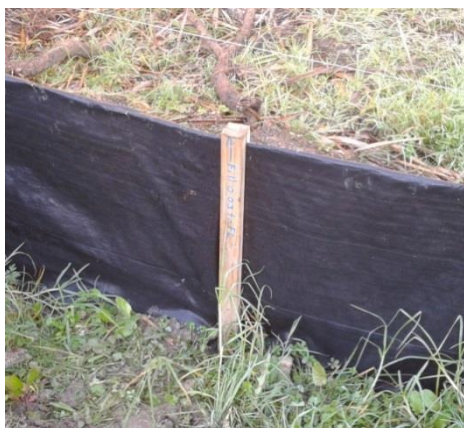
Figure 80: Silt fence joins. Left hand photo shows battens used to join the lengths. Right hand photo shows doubling over of fabric at end around the waratah
