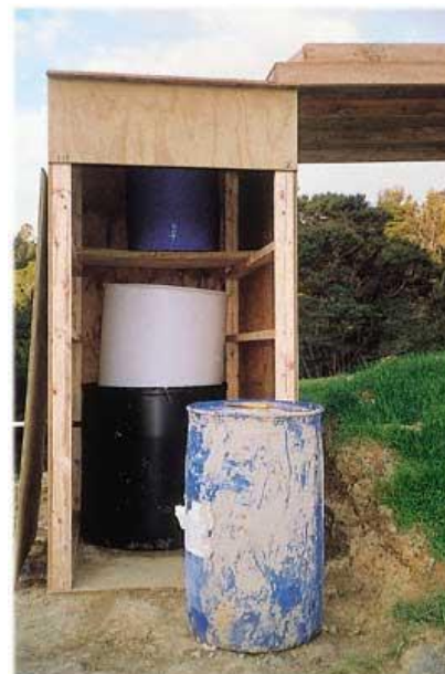
Figure 99: rainfall activated flocculant treatment device
