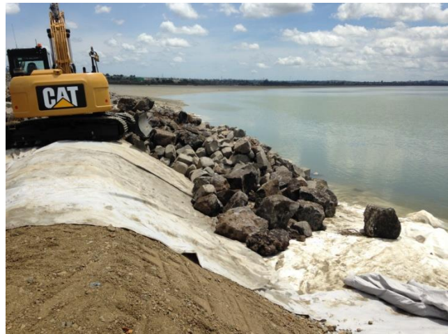
Figure 133: Use of geotextiles and coastal protection rock
