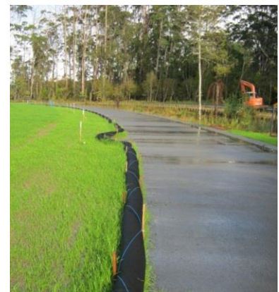
Figure 95: Silt sock used to provide control during final landscaping works
