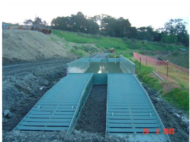
Figure 37: Example of a shaker ramp
