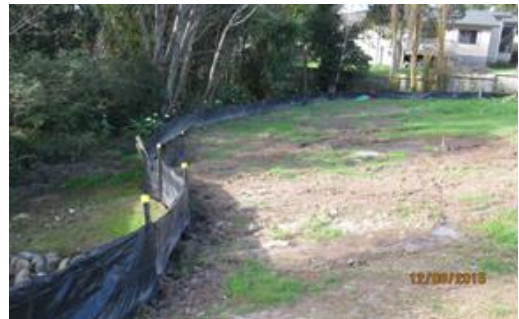
Figure 107: Silt fence
