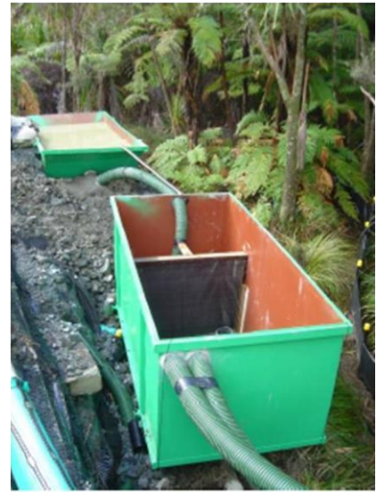
Figure 104: Dewatering skip bin
