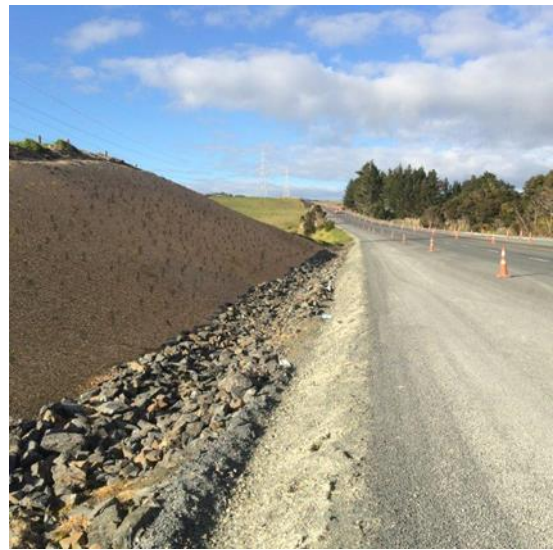
Figure 56: Woodchip to stabilise the finished batter slope
