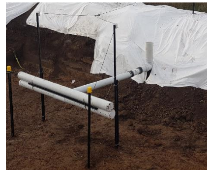
Figure 77: Decanting earth bund system and close up of T-bar dewatering device.
