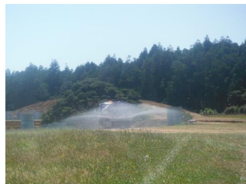
Figure 129: Regular wetting of the haul road
