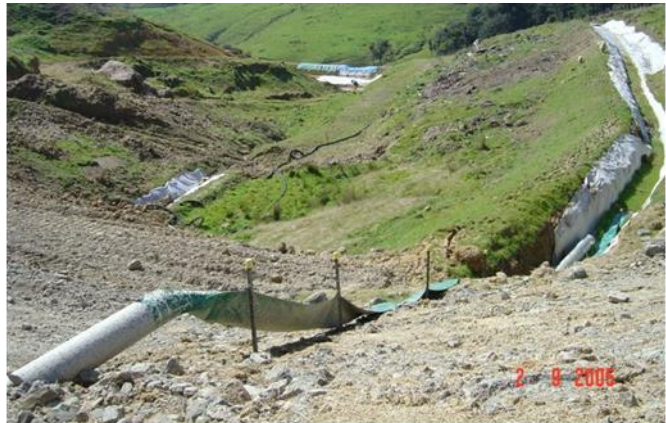
Figure 11: Flume installed to protect steep slope
