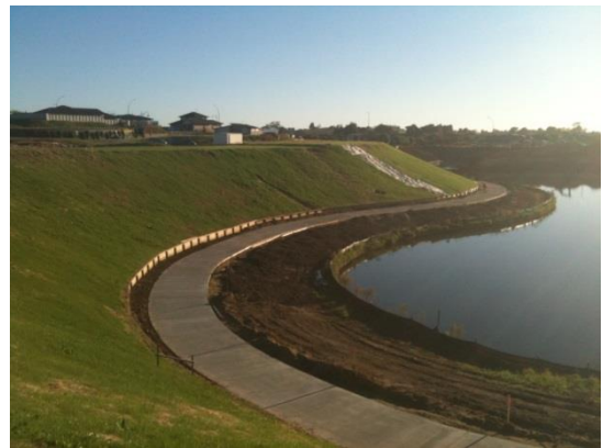
Figure 42: Grass stabilised earthworks site. Batter and building platforms
