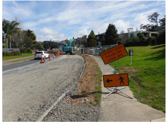
Figure 109: Use of stabilisation products and progressive stabilisation
