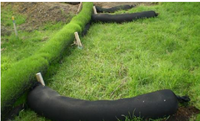
Figure 90: Compost silt socks with returns installed
