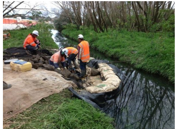
Figure 122: Sandbag coffer dam installed to complete stormwater outfall
