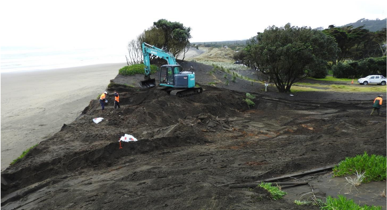
Figure 134: Dune reshaping
