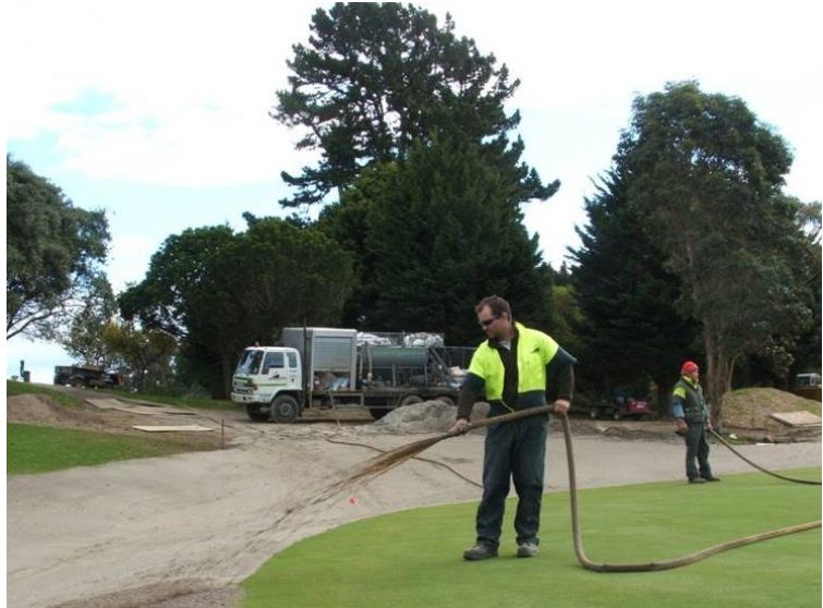
Figure 47: Specialist application of hydroseed
