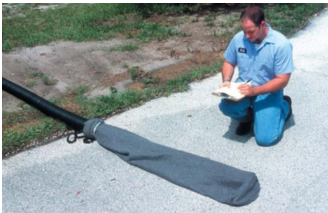
Figure 105: Dewatering bag and pipe sock
