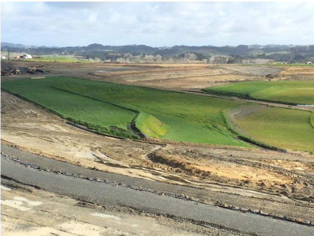
Good example of staged construction and progressive stabilisation
