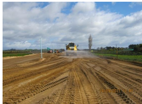
Figure 128: Water truck dampening down the works area
