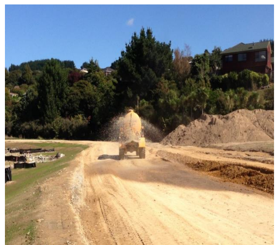
Figure 125: Dust suppression using a water cart
