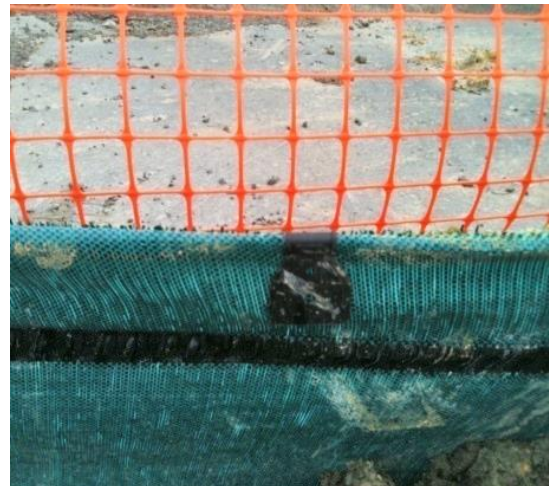
Figure 85: Use of silt fence clips
