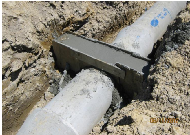
Figure 70: Example of an anti-seep collar
