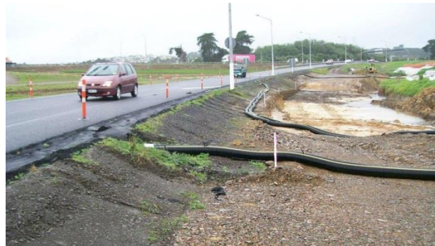
Figure 29: Flume conveying clean water over the works area
