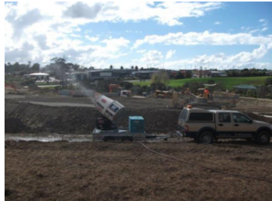
Figure 126: Snow blowing machine to provide dust control during a liming operation
