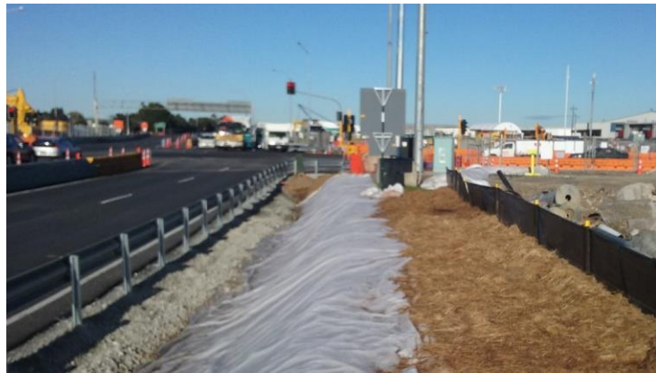
Figure 108: Progressive stabilisation in limited space
