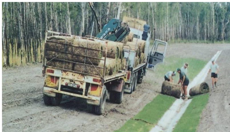
Figure 51: Turf being placed adjacent to a stabilised swale
