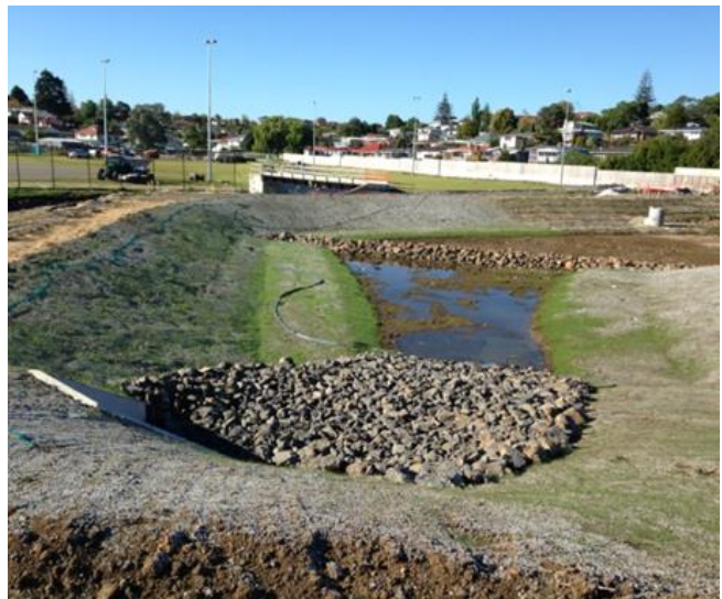
Figure 49: Recently applied hydroseed on a stormwater wetland
