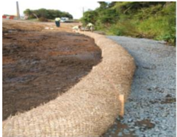
Figure 89: Silt sock used to provide control during final landscaping
