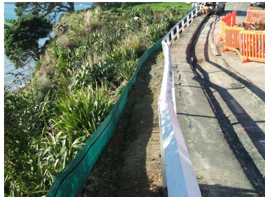
Figure 79: Silt fence installed on edge of works
