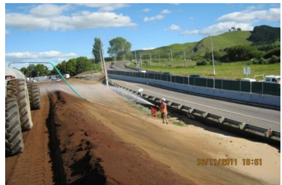
Figure 127: Dust suppression using soil binders/polymers
