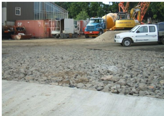
Figure 34: Stabilised entranceway
