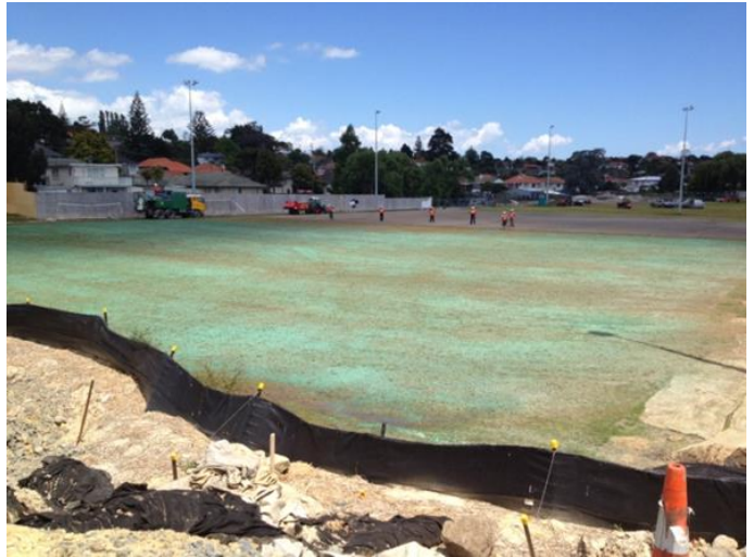
Figure 48: Sports field being hydroseeded. Sediment control remains installed until an 80% grass strike has established
