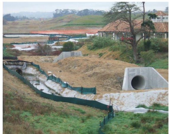
Figure 117: Examples of temporary stream diversion installed to allow permanent culverts to be installed off-line
