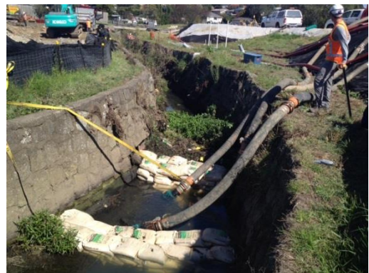
Figure 116: Commencement of over pumping to allow for in-stream works
