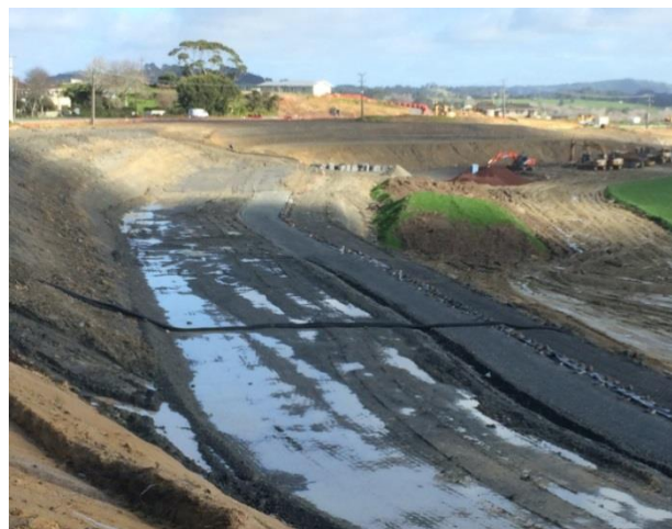
Figure 33: Pipe-drop structures conveying upper water down an exposed slope
