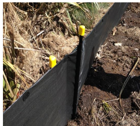
Figure 80: Silt fence joins. Left hand photo shows battens used to join the lengths. Right hand photo shows doubling over of fabric at end around the waratah
