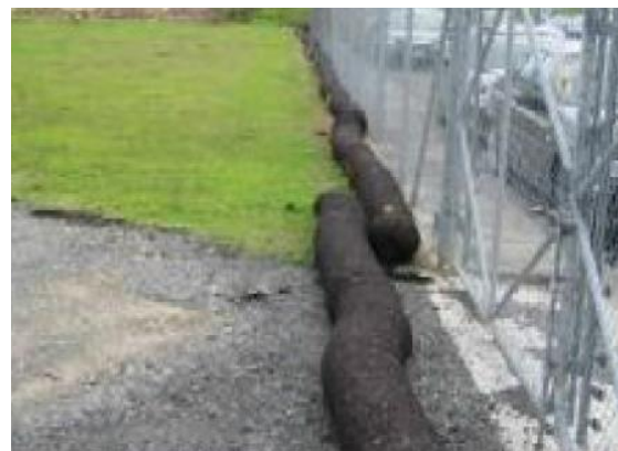
Figure 91: Silt sock with 1 m overlapping joint
