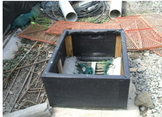
Figure 96: Stormwater inlet protection silt fence within a construction yard
