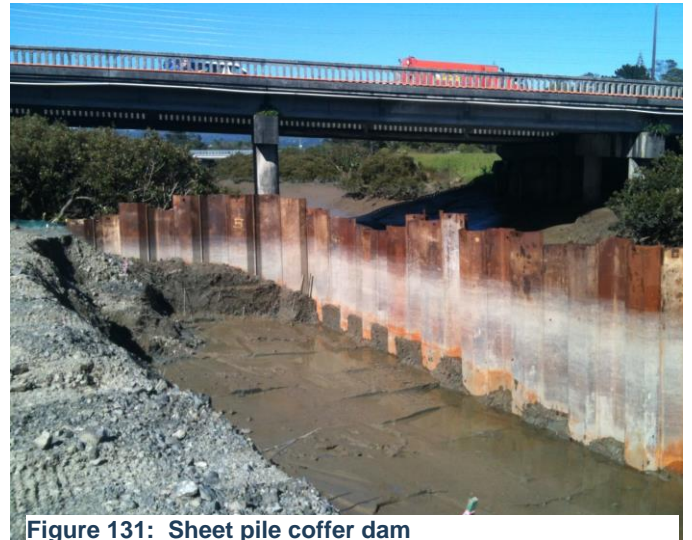
Figure 131: Sheet pile coffer dam
