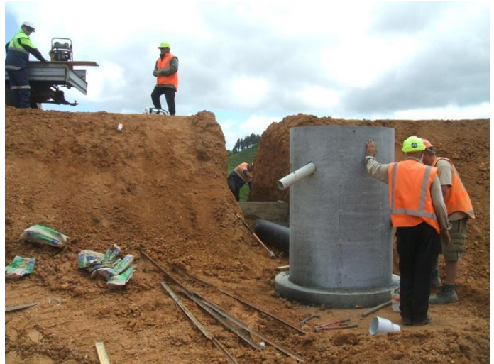
Figure 74: Installation of the outlet pipe and the anti-seep collars
