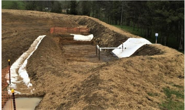
Figure 77: Decanting earth bund system and close up of T-bar dewatering device.
