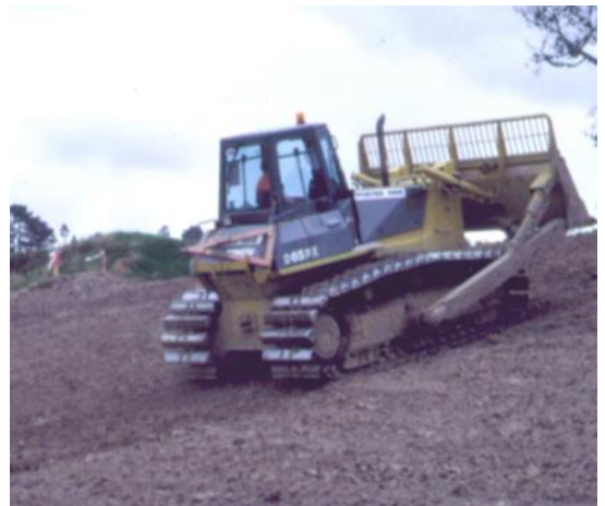
Figure 38: Surface roughening with bulldozer
