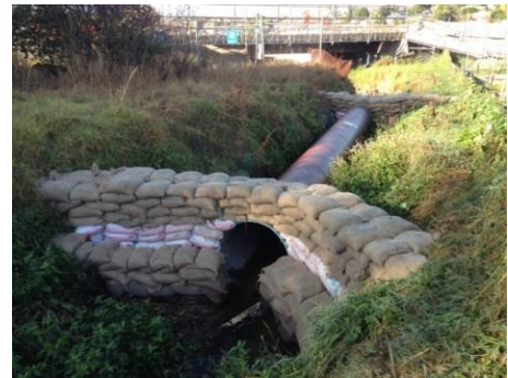
Figure 114: In the process of constructing a temporary crossing
