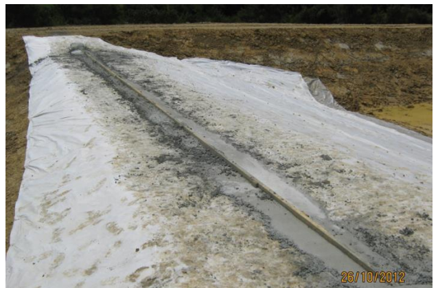
Figure 68: Example of a level spreader
