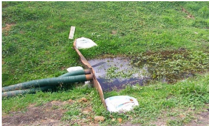
Figure 115: Water being diverted past a construction works area
