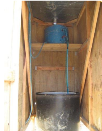
Figure 102: Header tank
