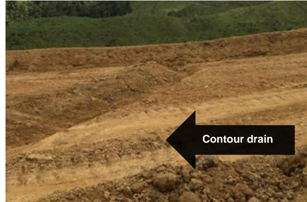
Figure 21: Contour drain
