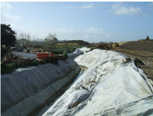
Figure 117: Examples of temporary stream diversion installed to allow permanent culverts to be installed off-line
