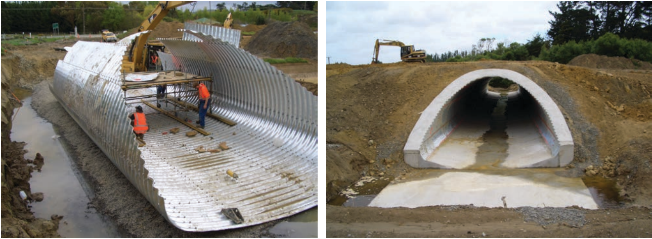
Galvanised steel corrugated multiplate culvert underpass under construction
