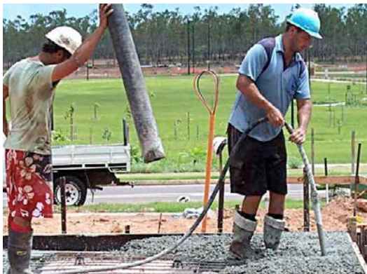
Figure 12: Immersion poker vibration
