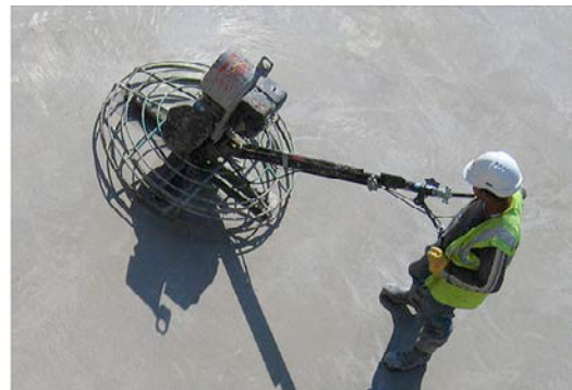
Figure 16: Power floating
