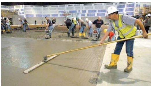
Figure 13: Ball floating
