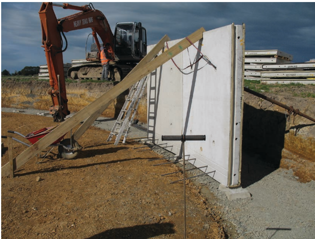
Storage tank, precast reinforced concrete panel construction
