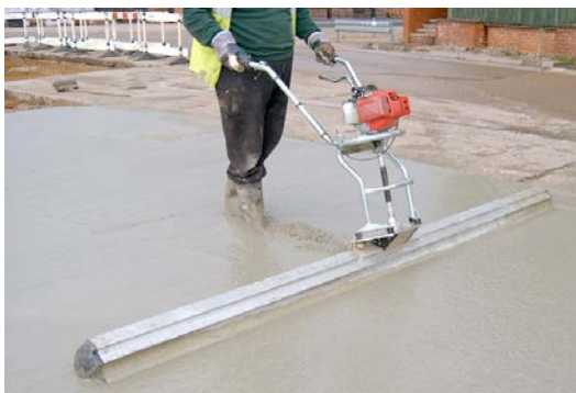
Figure 11: Lightweight vibrating screed
