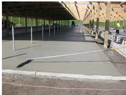
Figure 15: Grooving tool
