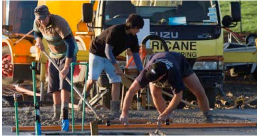
Figure 10: Hand tamping
