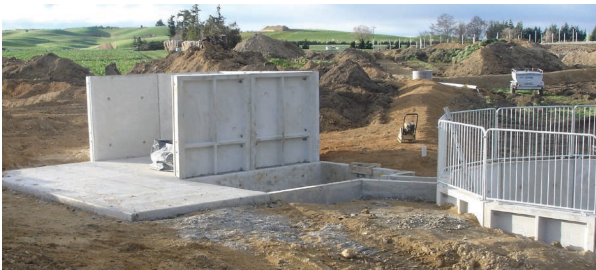
Reinforced concrete storage bunker with draining pad, stone-trap and sump
