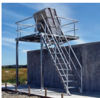
Slope screen with platform and safety railing, access ladder at rear
