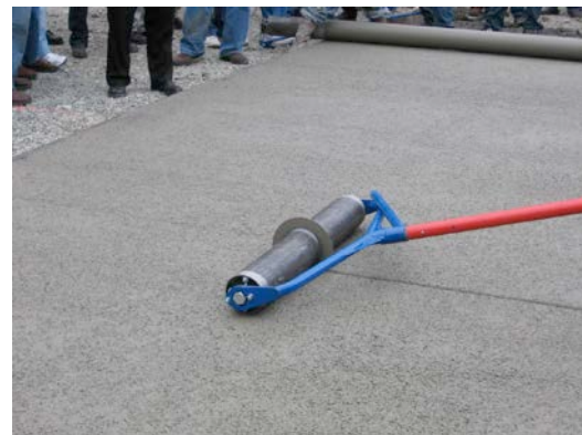
Figure 18: Jointing tool or T section
