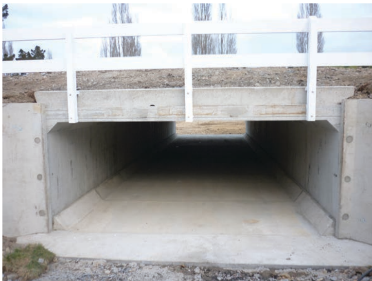
Box culvert underpass near completion
