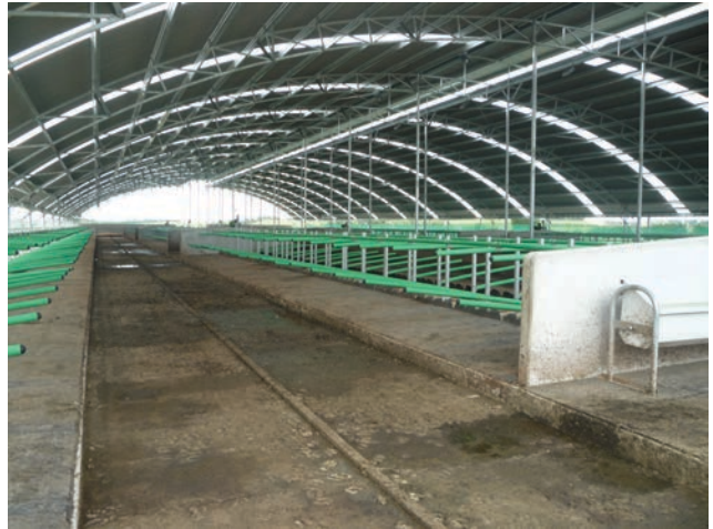
Covered feed pad
