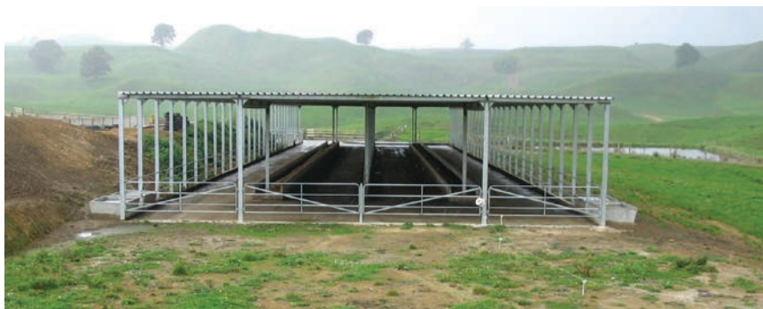
Covered feed pad
