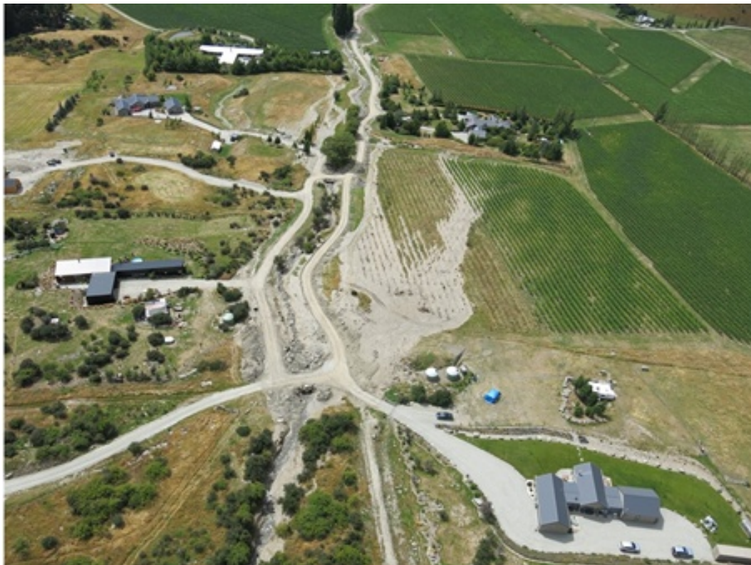
Figure 7. View north down Tussock Creek subdivision (Gibbston Valley) showing sediment deposited in and around the channel, and across part of a vineyard. Much of the sediment blocking the creek had been cleared at time of photo (12 th February 2020, photo ORC).
