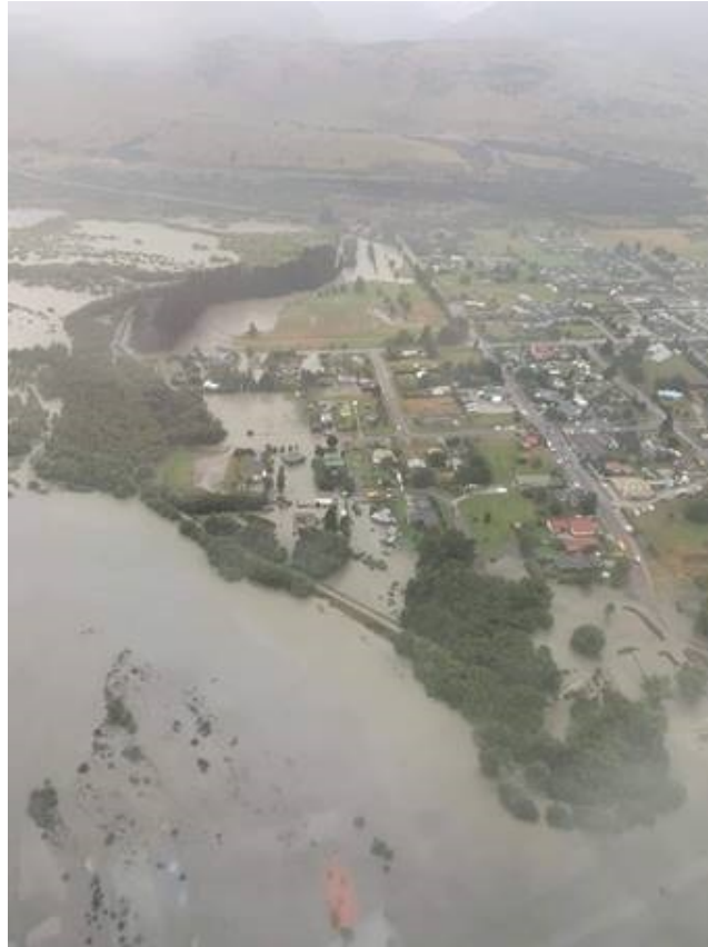
Figure 6. Flooding in Glenorchy, 4 February 2020 around 6.30pm. Rees River Delta in the foreground and Lagoon to the left of the photograph (photo: Luke Hunter, Done Rite Contracting Ltd)
