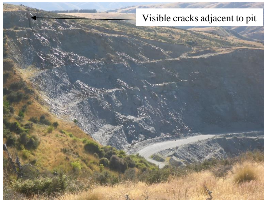
Figure 2. Photo looking across Deepdell South Pit to the rock mass with the vertical cracks.
