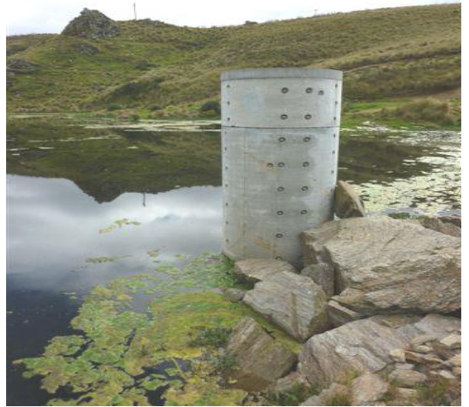
Plate 6. Typical Silt Pond Decant Structure
