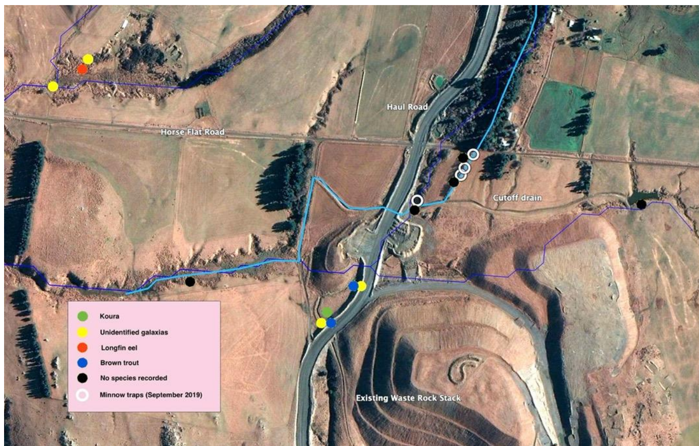
Figure 15 Aerial map showing the location of the modified watercourse adjacent to the haul road described in section 5.1.1. The thick light blue line indicates the watercourse flow path from top of the aerial down to the left towards Camp Creek (piped under the culvert). The finer dark blue lines are imported REC shape files. Note that fish and koura records for the tributary running through the middle of the map pre-date (1991-1987) the existing haul road and adjacent waste rock stacks.
