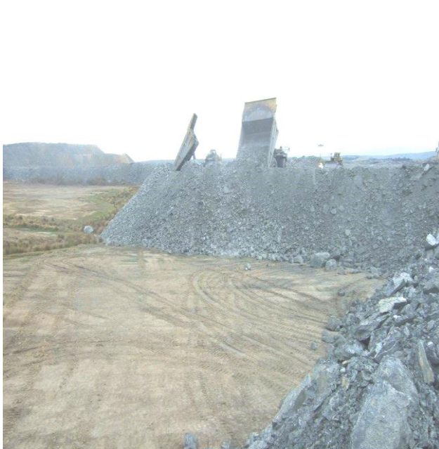
Plate 7. Rock Stack Tip Face (initial lift)
