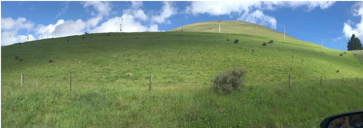
Figure 12. Typical backfill surface is smooth and has absence of gully features or tall tussock. Here, scattered Matagouri has established into pasture on an overburden embankment and if encouraged, could help enhance landscape (and easier to establish than tussock).
