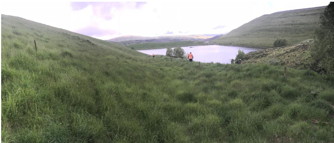
Figure 11. Rehabilitated and grazed 3:1 slopes (left) and 2:2 slopes (right, with benching) on either side of the fresh-water storage dam with planted willows (the tussock outcrop with non-native pines is a natural landscape). Resource consent conditions now specify neither pines nor willows (or alders or larches) are allowed to be planted (these should be replaced with native species over time).
