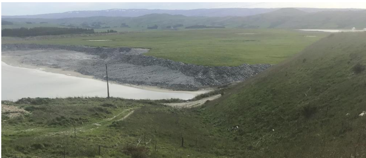
Figure 3 Tailings dam with partly rehabilitated cap supporting pasture. Note the three shallow ponds amid pasture on the backfill which may provide or supplement a suitable stock water supply, or be suitable locations for red tussock ( Chionochloa rubra ) establishment.
