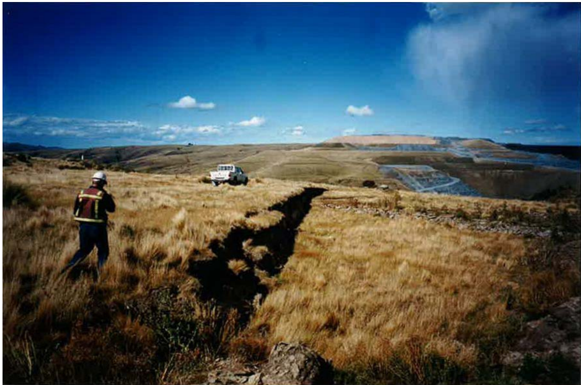
Photograph 1: View of failure head scarp looking south
