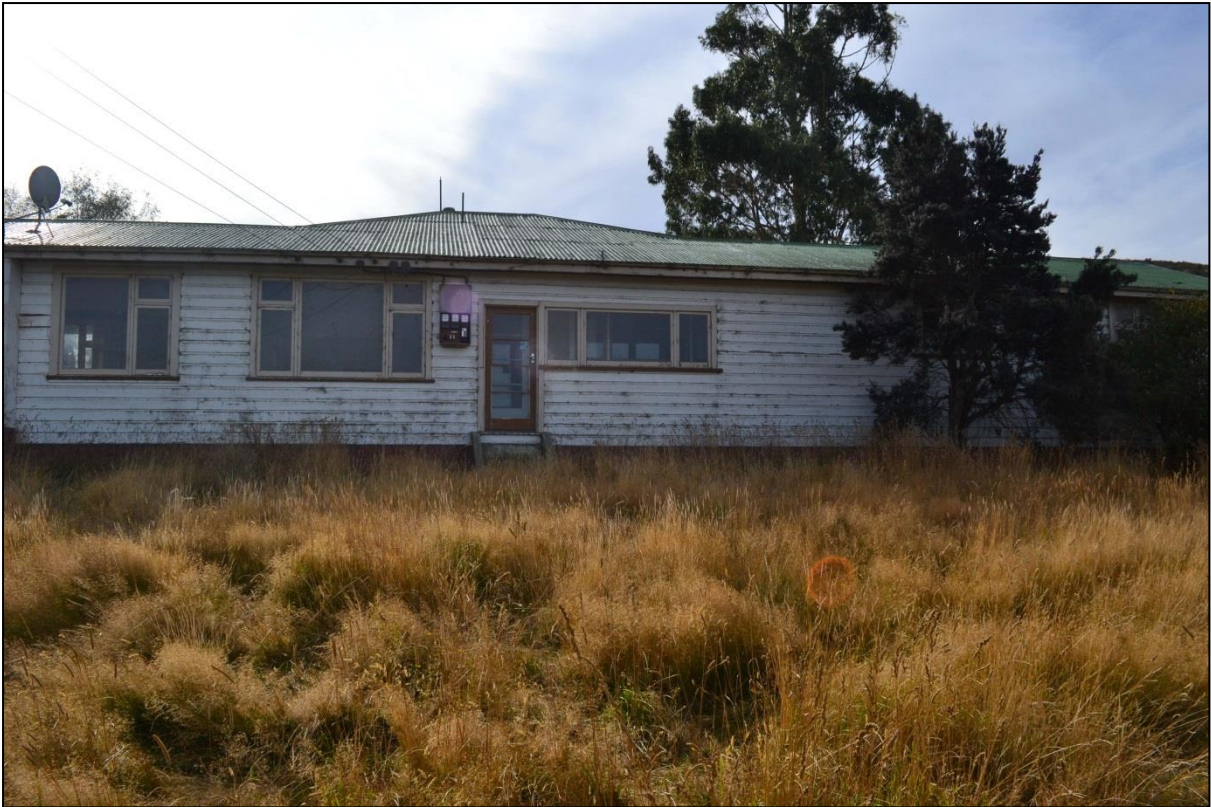
Figure 18. Front of modified villa looking north.
