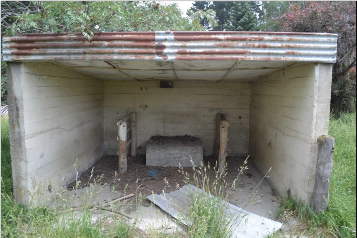
Figure 21. Concrete auxiliary building next to Horse Flat Road.
