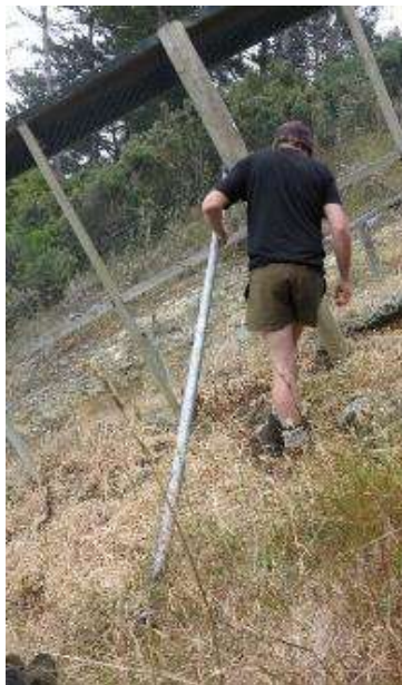
Figure 3-3 Eiger Section - Steep ground
