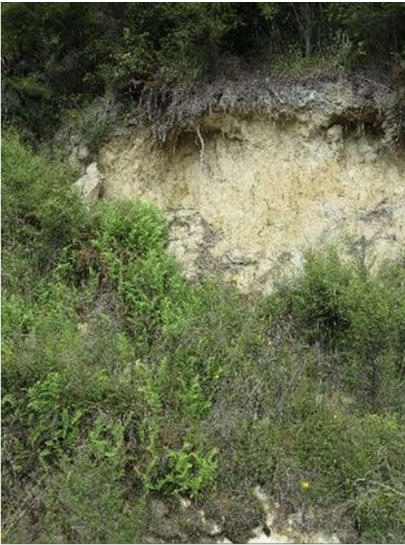
Figure 3-5: Upslope bank collapse (minor)
