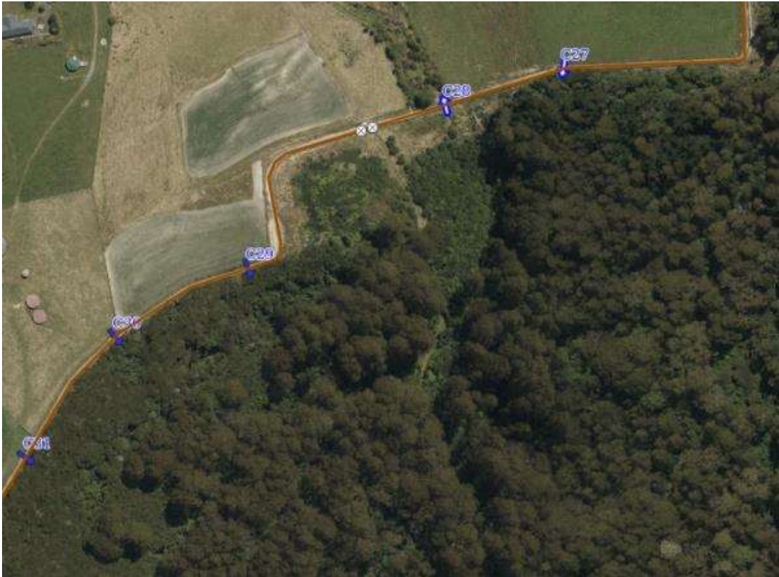
Triple Culvert Section
