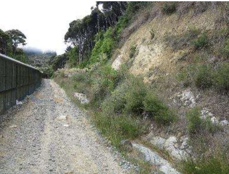
Figure 3-6: High cut slopes
