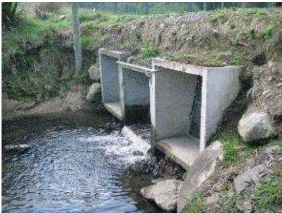
Triple Culvert Outlet
