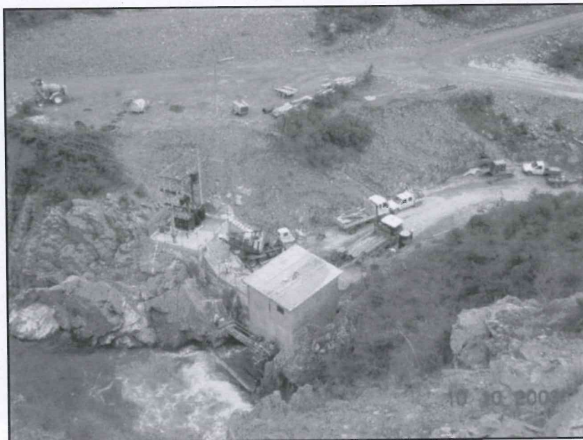
The new power house under construction in 2003.
