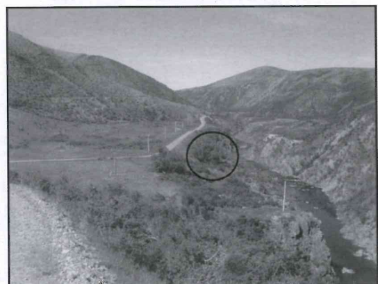
The same flat area today. On the right of the road the rear willow trees are located around the foundations and chimneys of the two houses, which are the last remnants of the construction camp.
