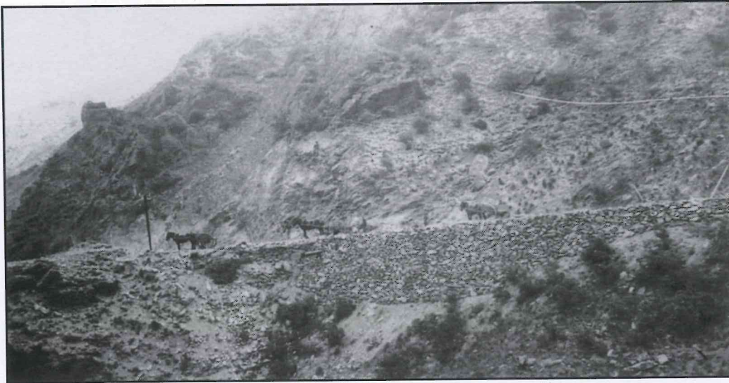
Horse and carts transporting rock from the right abutment quarry to the dam. A roadway has been made with rock quarried from the hillside.
