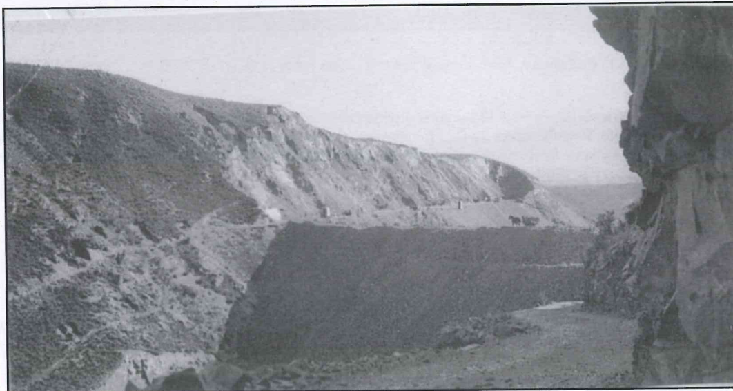
Horse and carts transporting rock from the right abutment quarry to the dam. A roadway has been made with rock quarried from the hillside.
