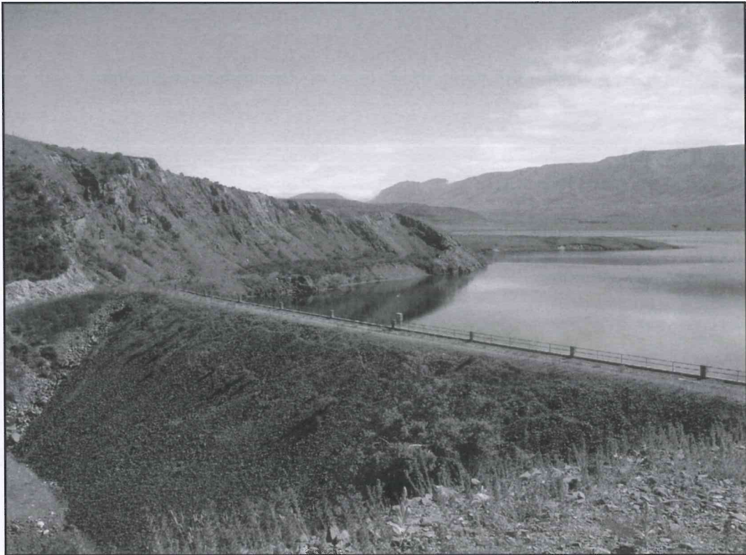
A recent view of the downstream face of the dam with the old quarry along the right abutment. Beyond the lake, at the rear, is the Hawkdun Range.
