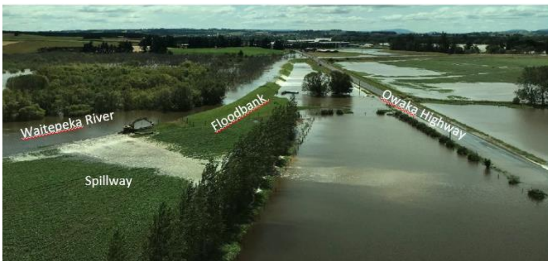
Figure 5. Waitepeka floodbank overtopping during February 2020 flood event.
