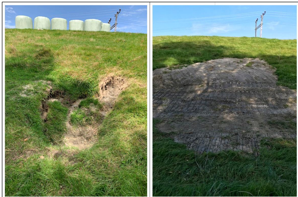
Figure 4. Main Balclutha stopbank (location 1, Figure 3) before (left) and after (right) repair.
