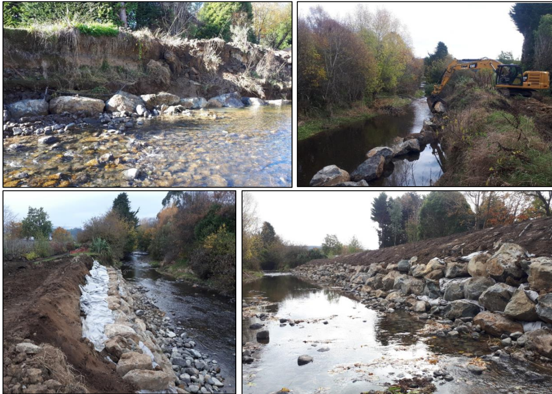
Figure 7. Waitati River Bank – during repair, and completed May 2020.
