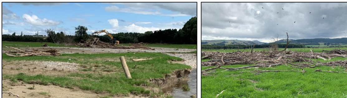
Figure 9. Removal of debris from Camperdown S-Bends, Upper Pomahaka River.
