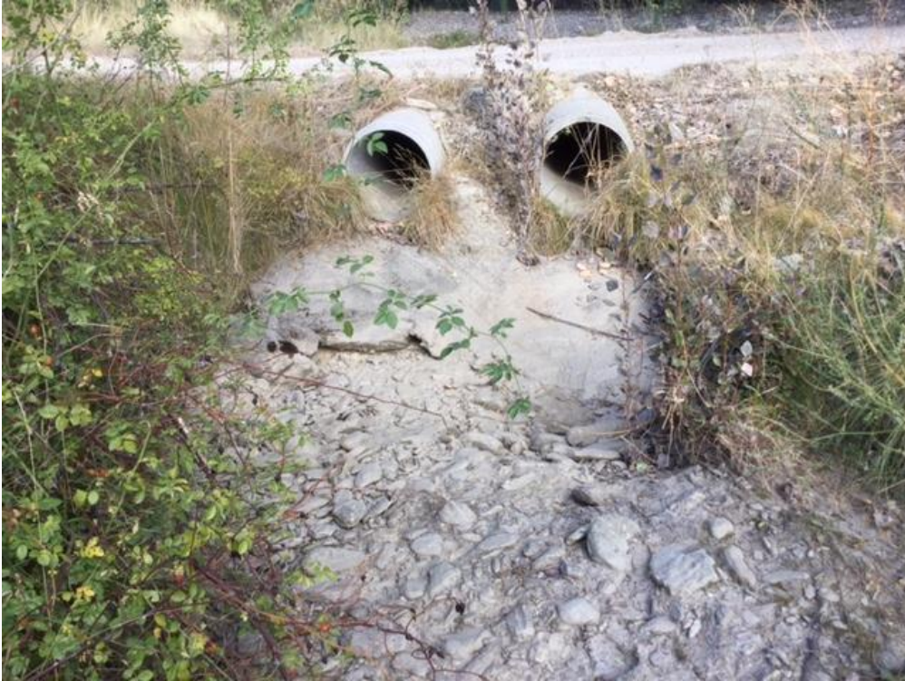
Figure 4. Black Quail culvert Friday the 24 th of March.
