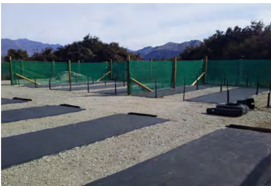
New plant beds in the expansion
