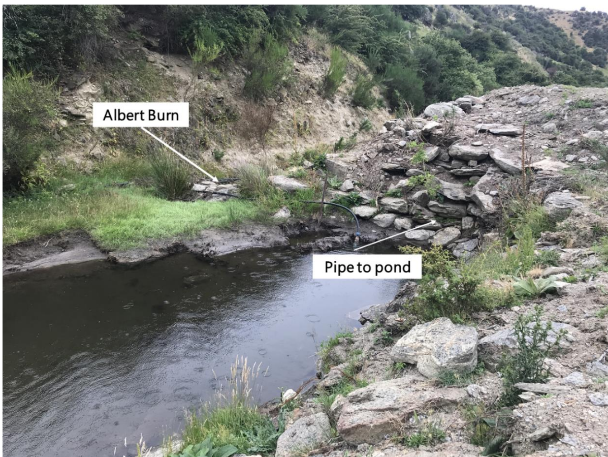
Figure 4: View downstream to the end wall of dam showing pipe to pond, and overflow to Albert Burn (January 2019).
