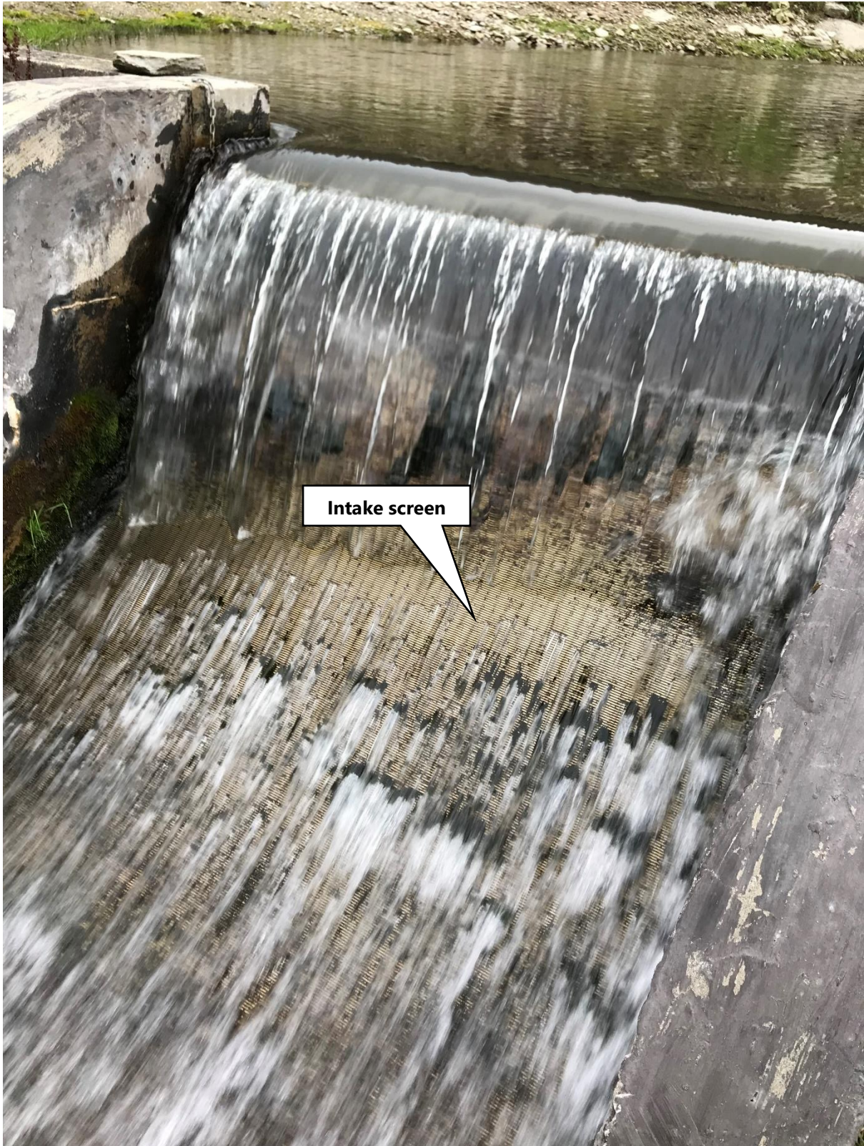
Figure 30: Albert Burn intake point behind fine-mesh screen (June, 2019)
