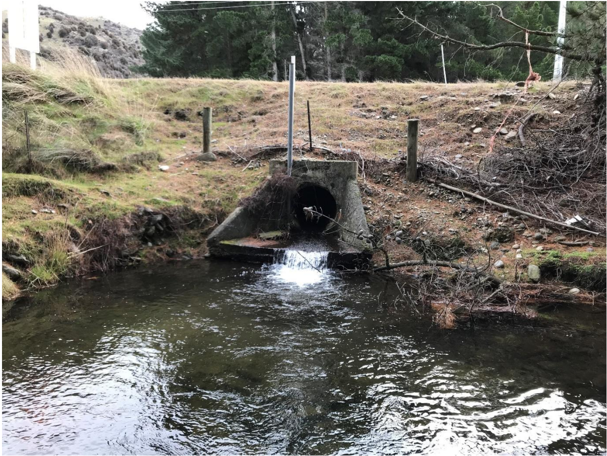
Figure 26: Schoolhouse Creek culvert under SH6 (July, 2019)
