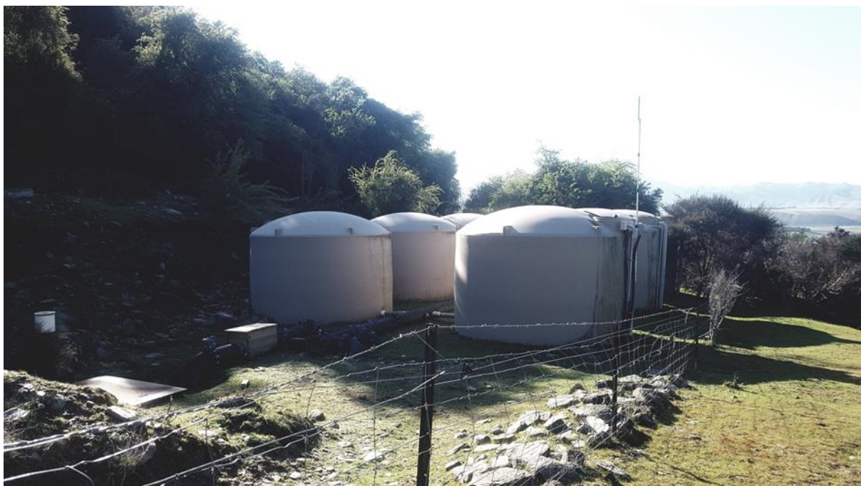
Figure 6: Tank farm where Albert Burn water is stored, and Clutha water can be stored if required (October 2018).
