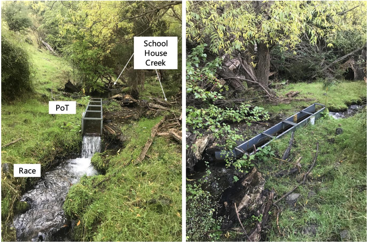
Figure 9: Schoolhouse Creek diversion to race with current infrastructure of a flume with staff gauge.
