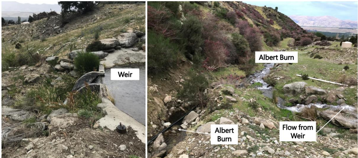
Figure 7: Left, weir at end of pond where diverted water flows back to the Albert Burn; right, view looking downstream from dam crest where the natural Albert Burn channel and overflow from pond converge (Left: January 2019, Right: June 2019).
