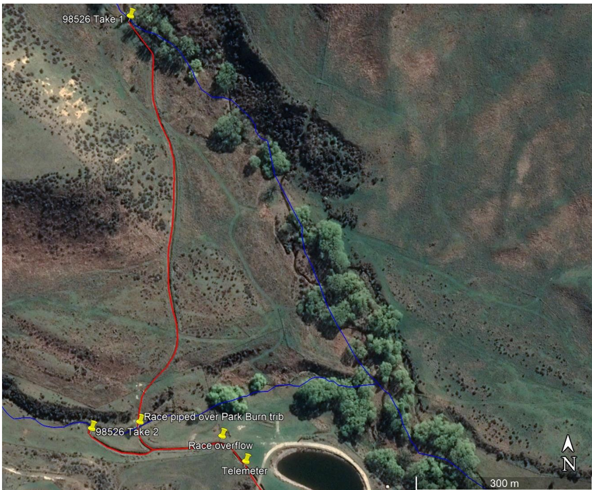
Figure 2: Close up of Rockburn water intake and conveyance infrastructure
