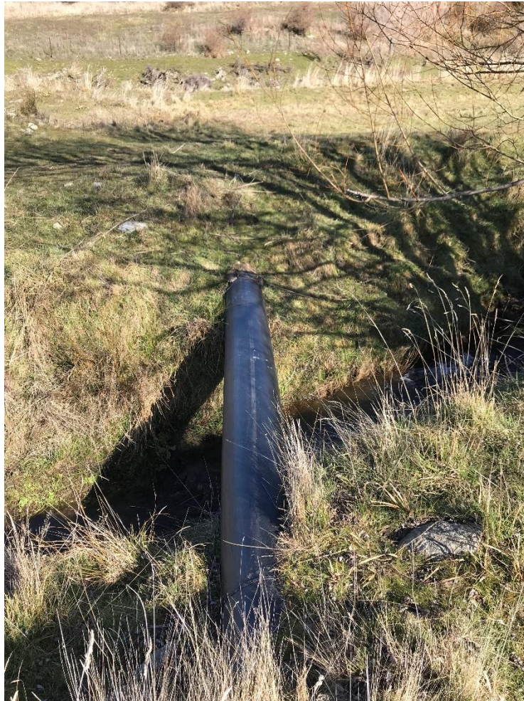
Figure 6: Rockburn main race piped across Park Burn tributary (August, 2019)
