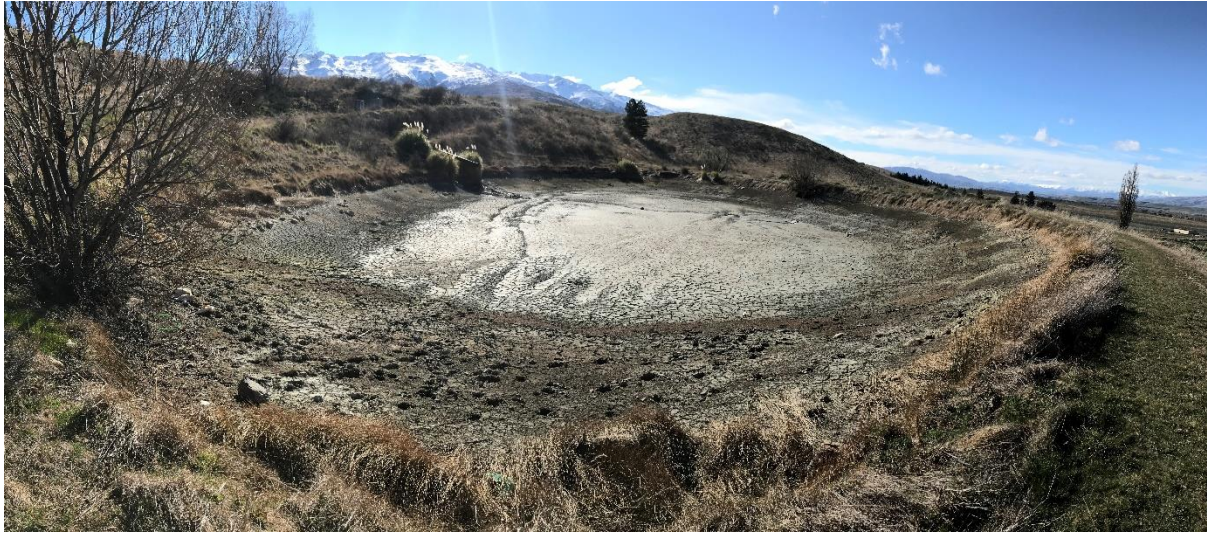
Figure 9: Rockburn Wines Ltd reservoir – empty to facilitate winter maintenance (August, 2019)
