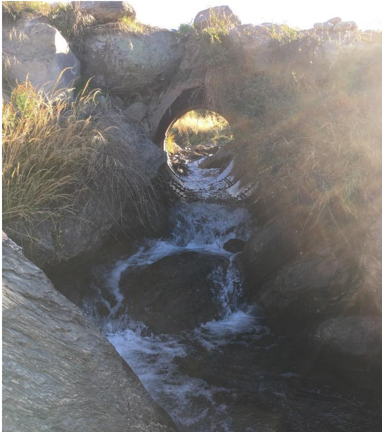
Figure 11: Amisfield Burn culvert on access track.
