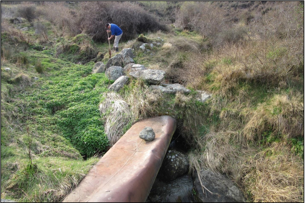
Figure 12: View of pipe across Sawyers Gully (September 2018)
