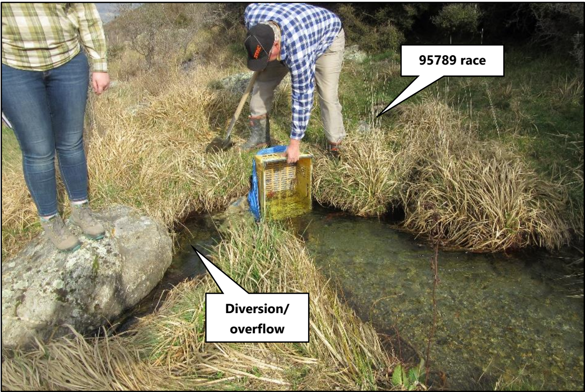
Figure 8: View of 9 Mile race flow control and diversion/overflow back to Amisfield Burn, approx. 40m downstream of intake (September 2018)
