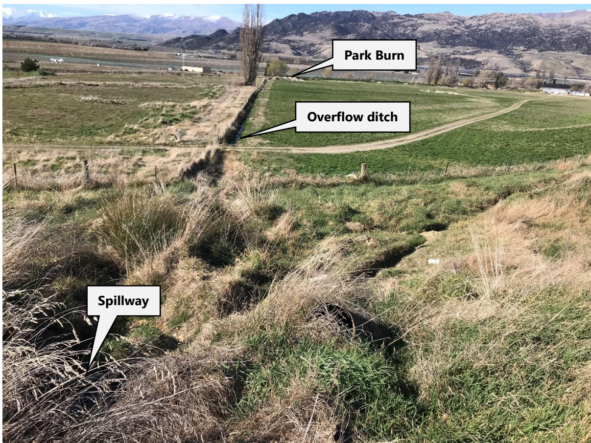
Figure 10: Storage pond spillway and overflow ditch, with the Park Burn in the background (August, 2019)
