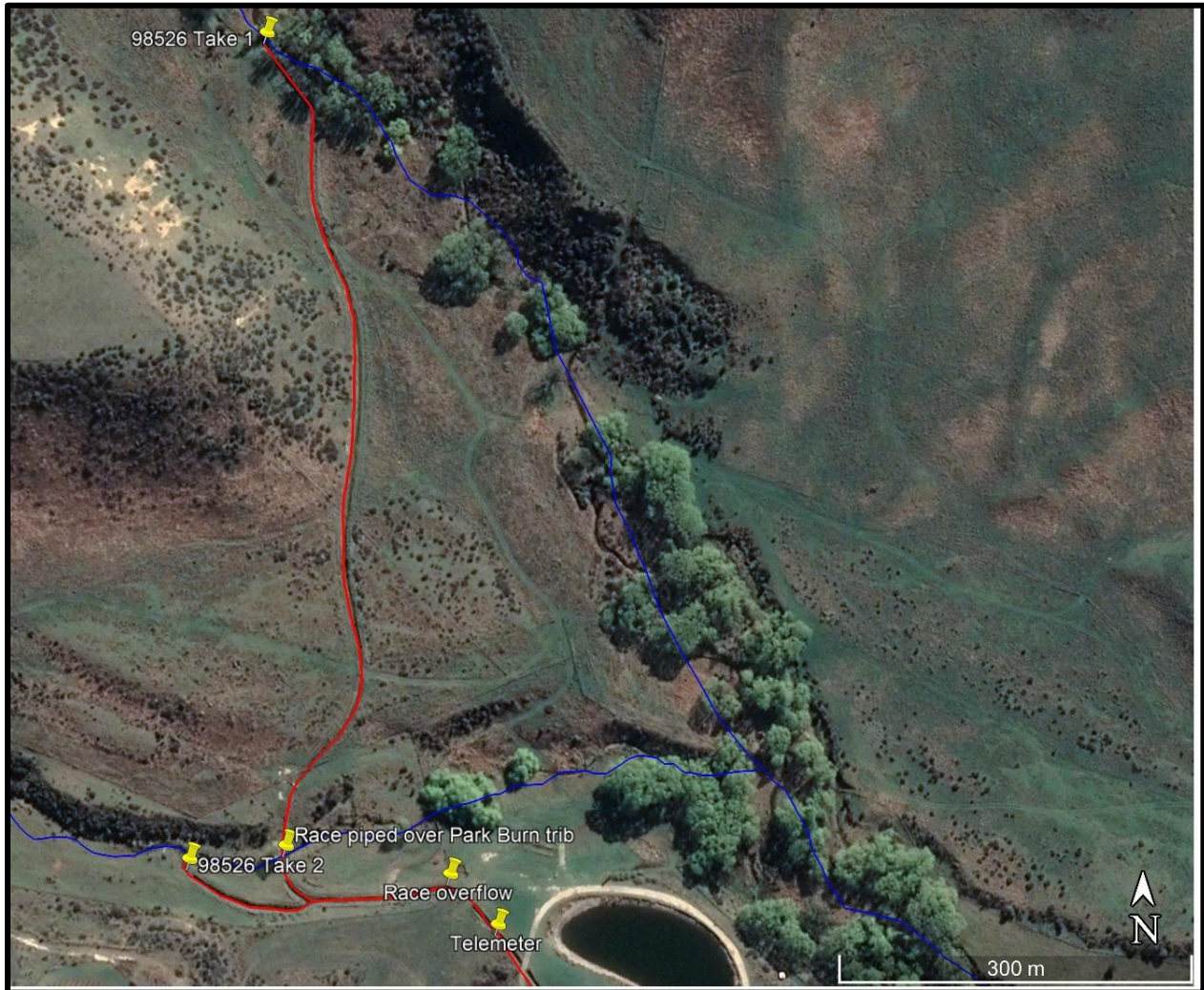
Image 2: Close up of Rockburn water intake and conveyance infrastructure (Source Application)
