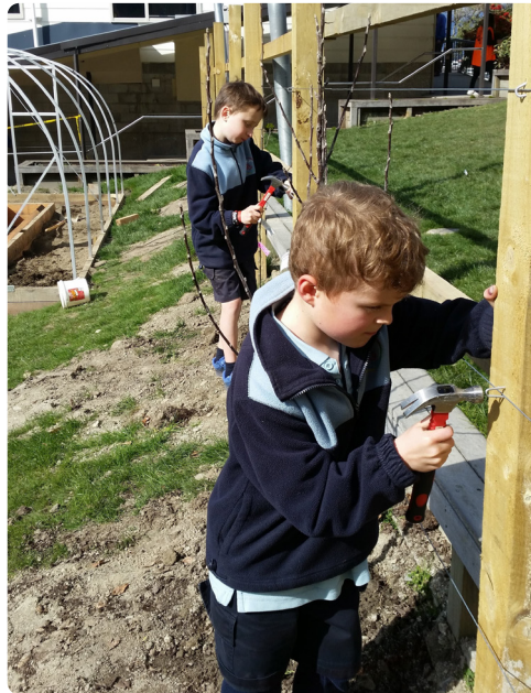
Building the fence above the garden
