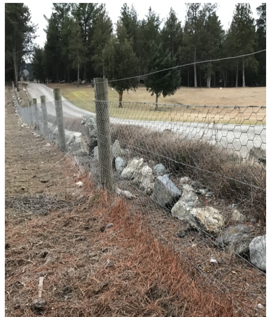
Rabbit proof fencing along the Clutha River edge, like this fence along the eastern hospital boundary, is one of the key long-term solutions.
