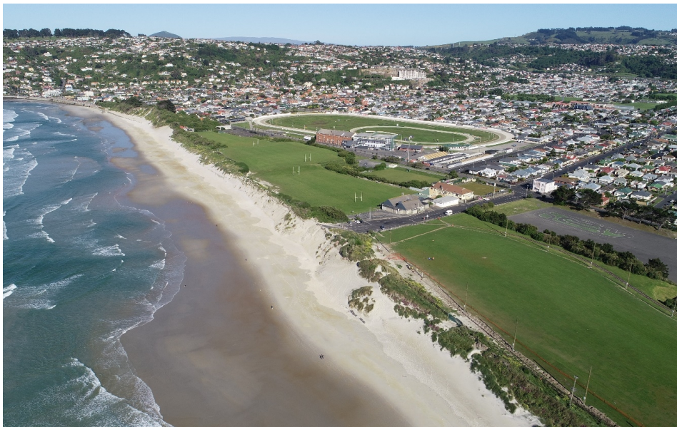
Figure 7. The Moana Rua dunes in front of Kettle Park (centre of image) form the seaward face of the closed historic landfill beneath the playing fields. DCC are currently exploring options for protection and adaptation in the area with projected sea level rise (St Kilda-St-Clair Coastal Plan). Photo credit Mike Hilton.
