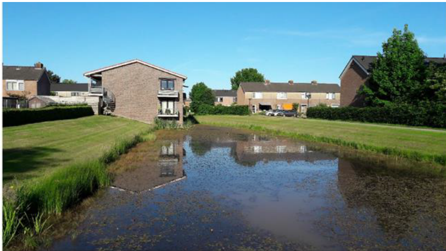
Figure 5. Greater New open canal dug during the district renovation of Oosterwolde-Zuid, The Netherlands: water storage, drainage, improved water quality and overall quality of the public space. (Golder Associates report on protection options for managing rising groundwater in South Dunedin to ORC (2017).
