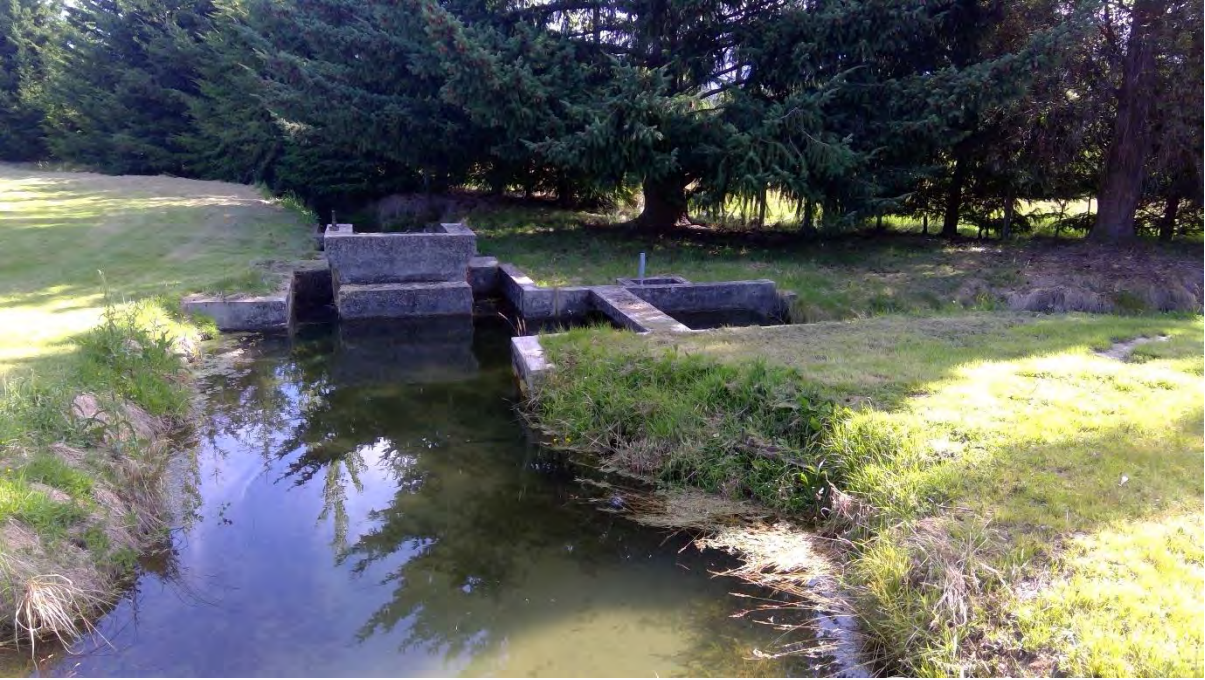
Plate 17: Weir on Mooney Road Pipeline
