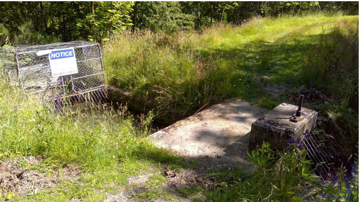
Plate 18: Junction Branch to Morven Ferry Pipeline
